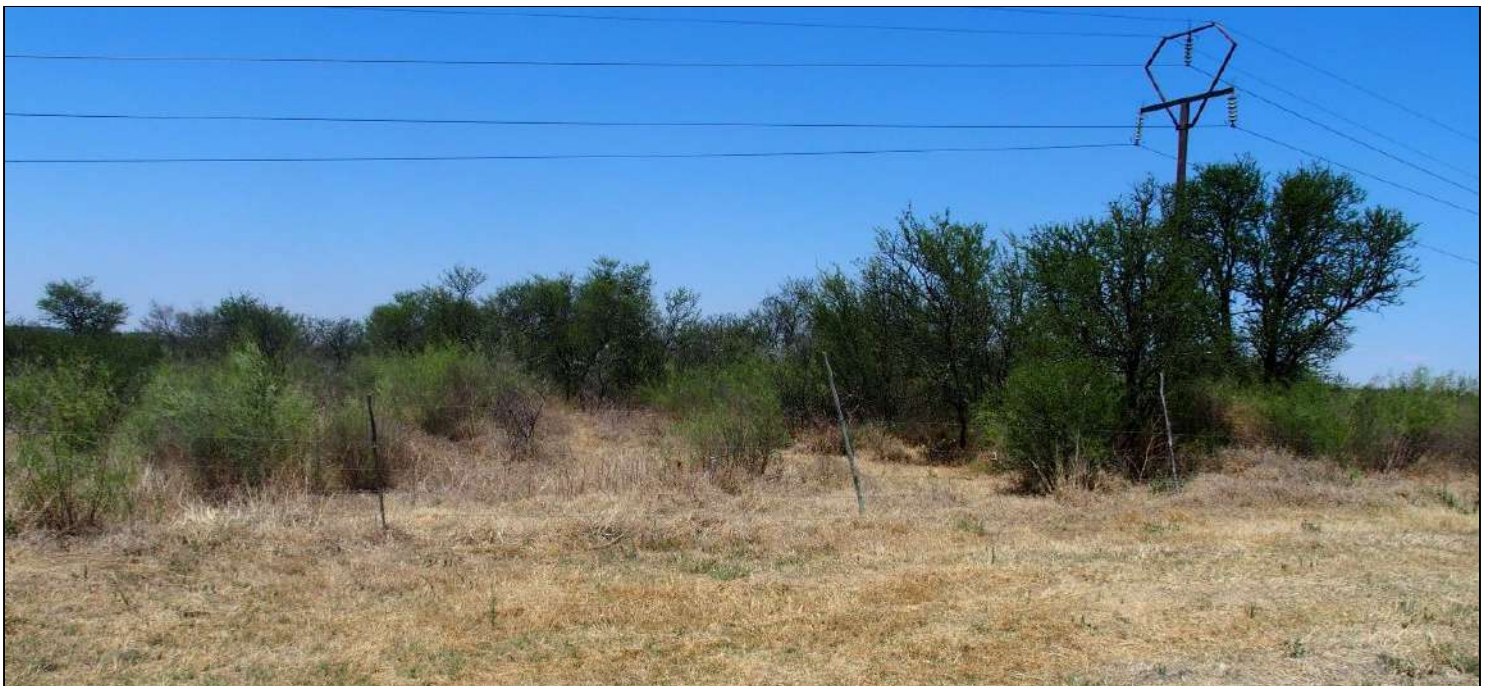
Figure 4.11 Looking East from the northern boundary of the Rondavel property at the point where the proposed power line would cross the river. Note the heavily compacted grass of the wide Rondavel farm fence-line track in the foreground and the major power line on the neighbouring farm to the east.
