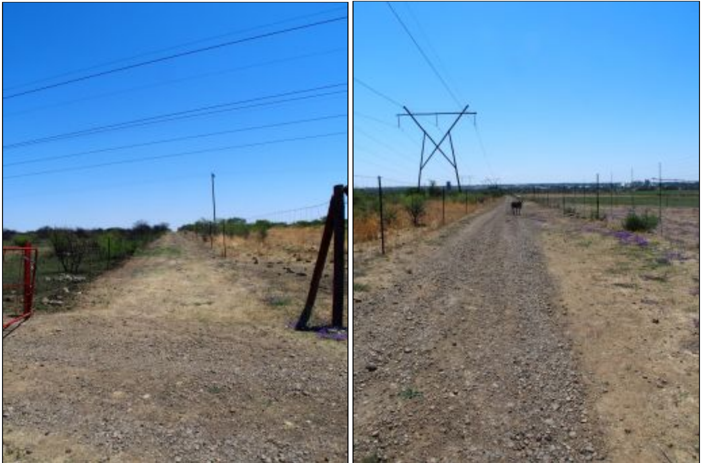
Figure 4.5: Along the Mid-East power line. Note the overgrazing on the farm track verge and grazed open grass in the field on the left. Also note the major power lines extending along the track.
