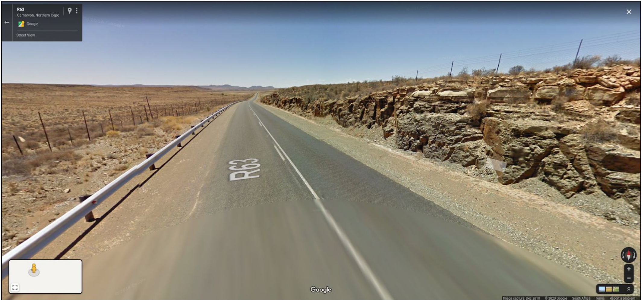
Figure 6.5 Contextual Images. Facing north towards Carnarvon along the R63 - Google Street View
