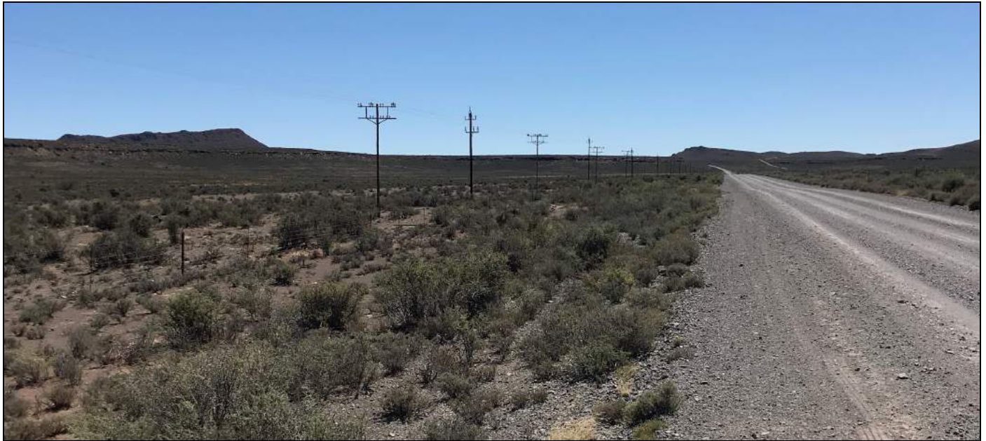
Figure 6: Existing overhead line that runs along the existing road
