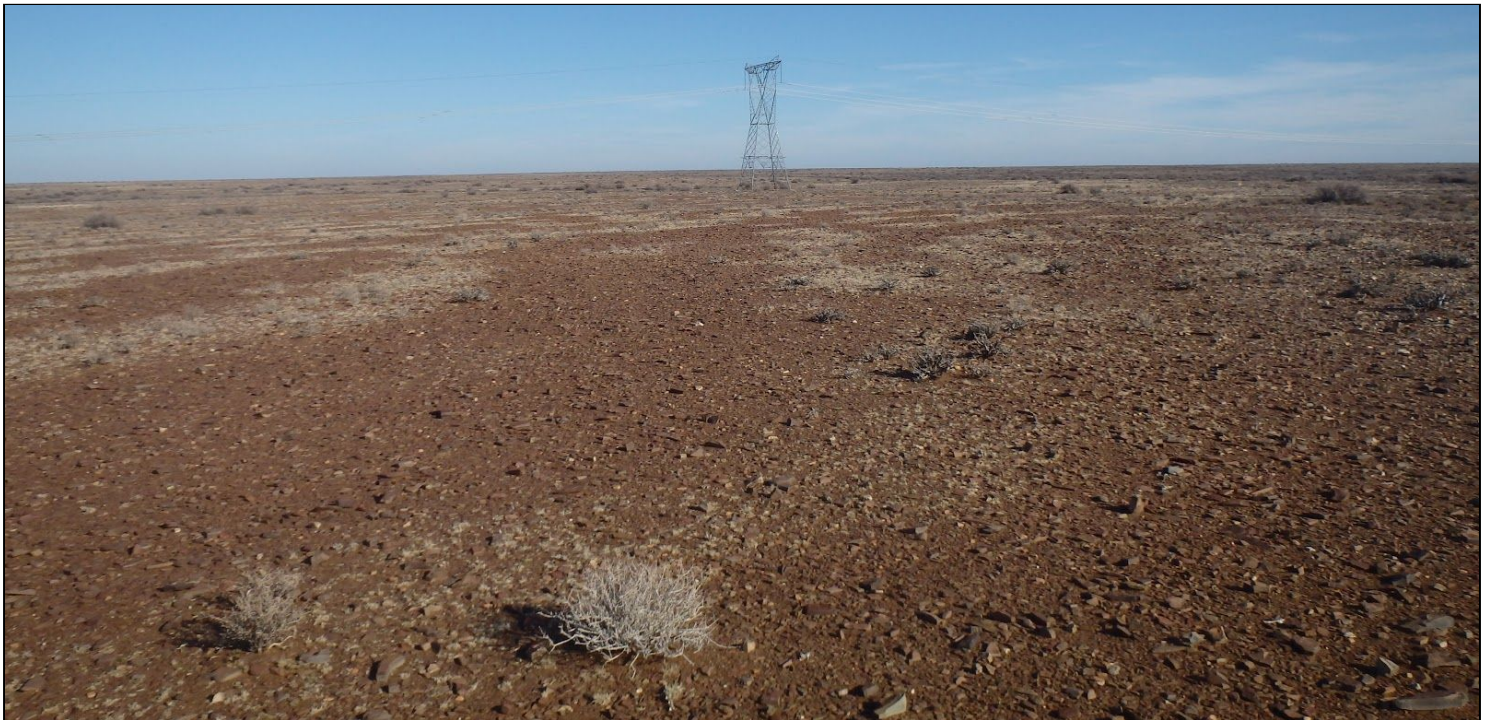
Figure 4.5: Overlooking KT PV4 from the southwest, note existing grid connection infrastructure
