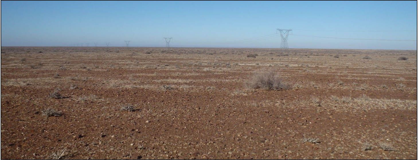
Figure 4.6: Overlooking KT PV4 from the southwest, note existing grid connection infrastructure
