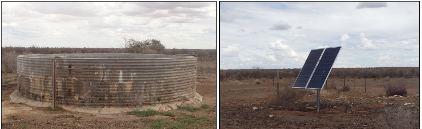
Figure 6.2: Concrete tank and kraal complex within KT PV1
