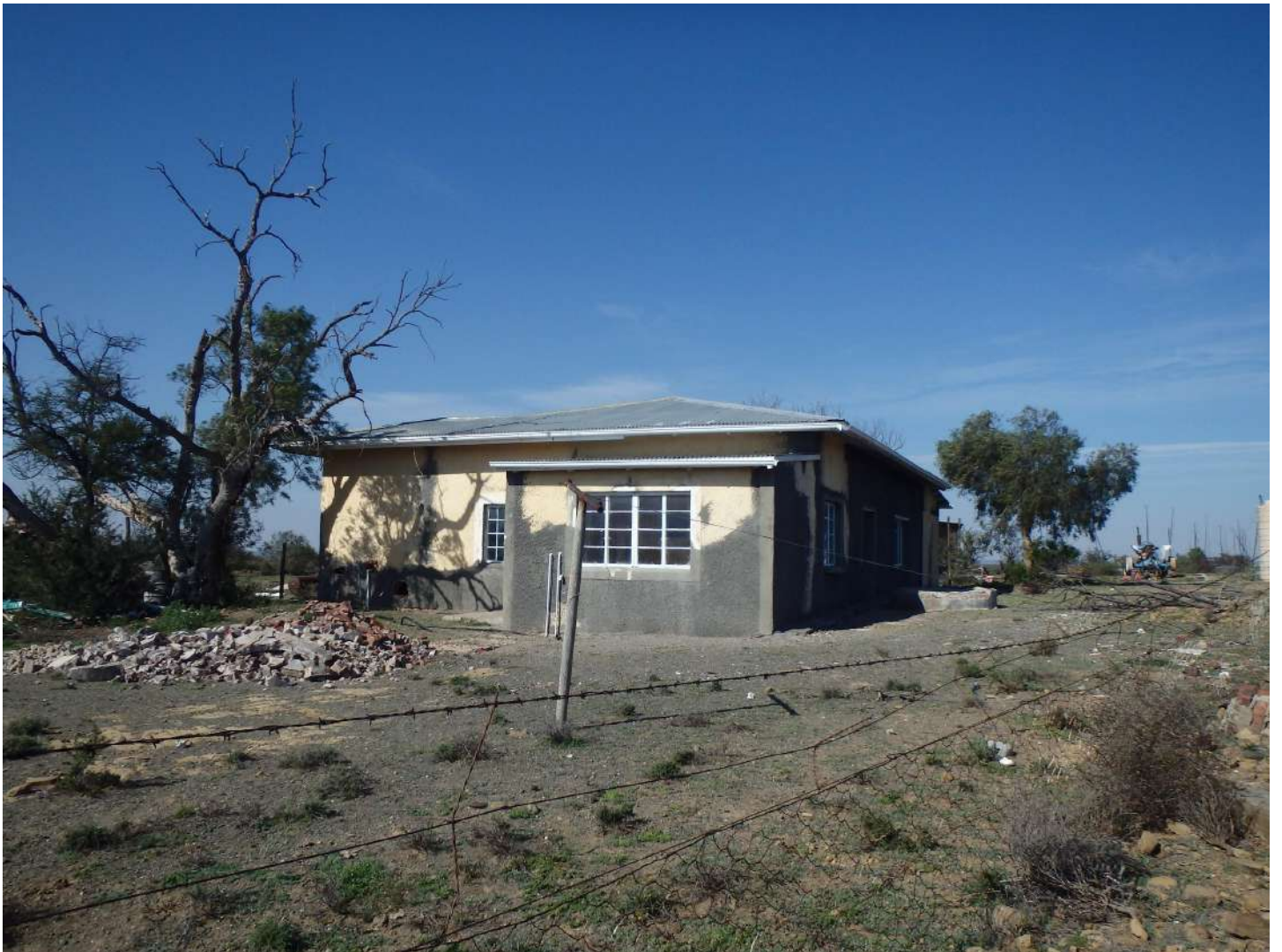
Figure 6.17: Observation ABD092 - Karroorivier Farmhouse complex, hipped corrugated iron roof
