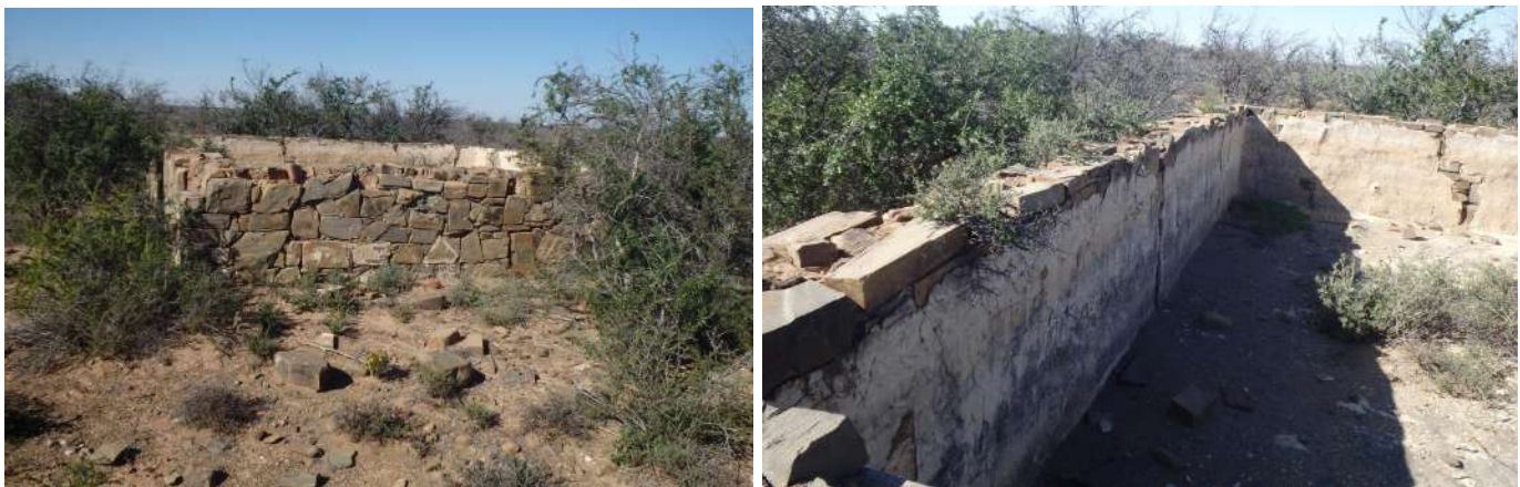
Figure 5.3 Observation ABD036 - Square sandstone ruined farm dam, metal drum, bullet casings, glass, ceramics
