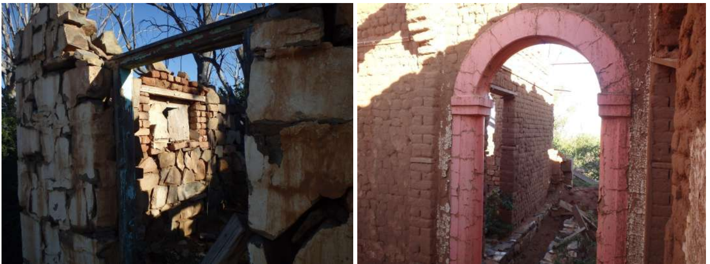
Figure 5.7: Observation ABD061 - Doornpoort ruined farmhouse complex
