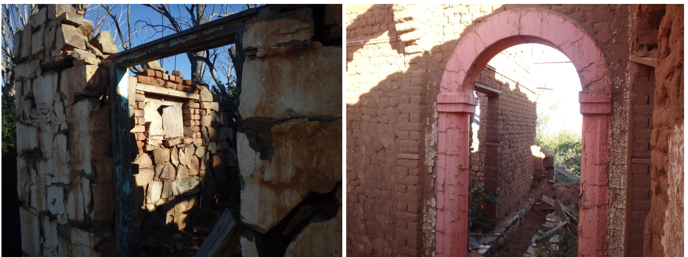
Figure 5.7: Observation ABD061 - Doornpoort ruined farmhouse complex
