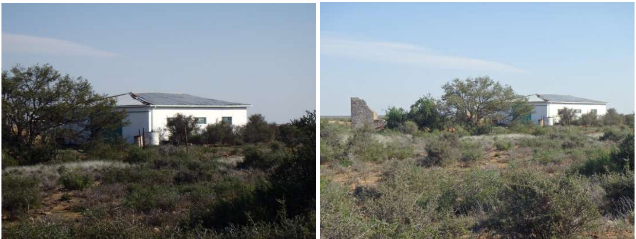
Figure 5.2: Observation ABD110 - Windermere farmhouse complex
