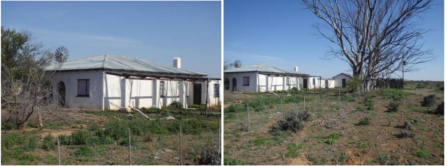
Figure 6.18: Observation ABD093 - Plaas 94, farmhouse complex, hipped corrugated iron roof, outbuildings
