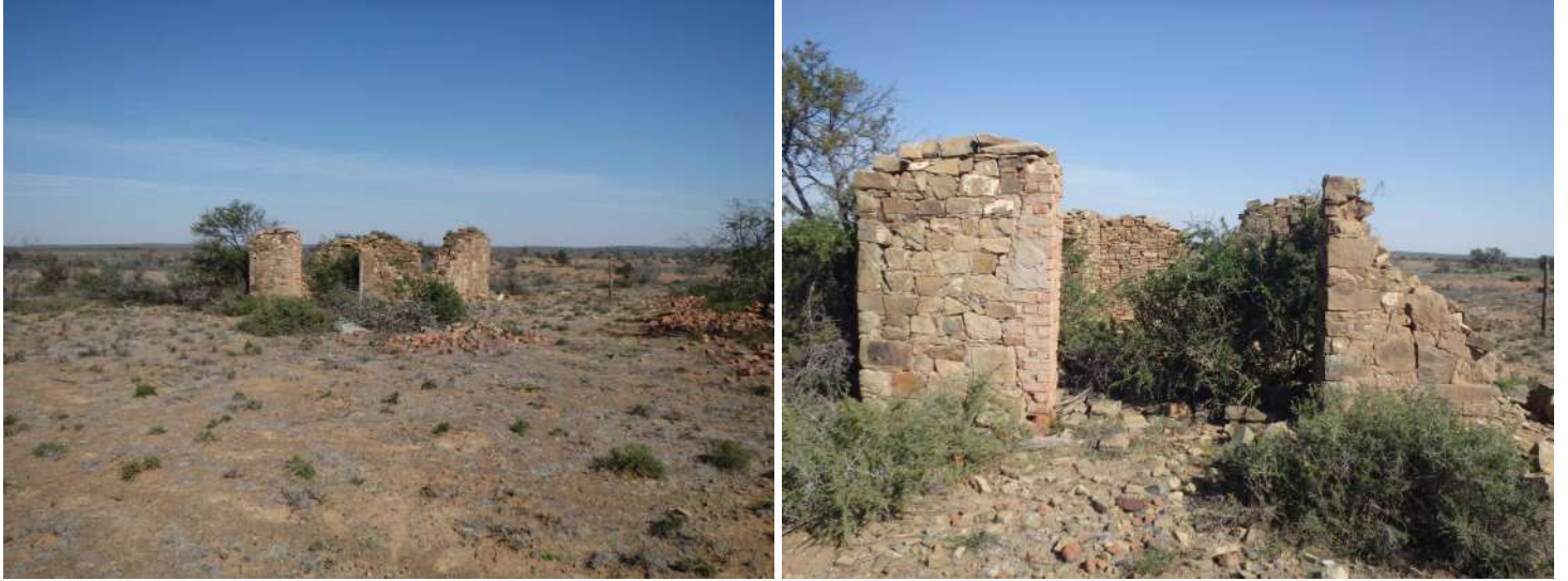
Figure 6.16: Observation ABD091 - Nooitgedacht Sandstone ruin, brick alterations, next to fully demolished brick buildings
