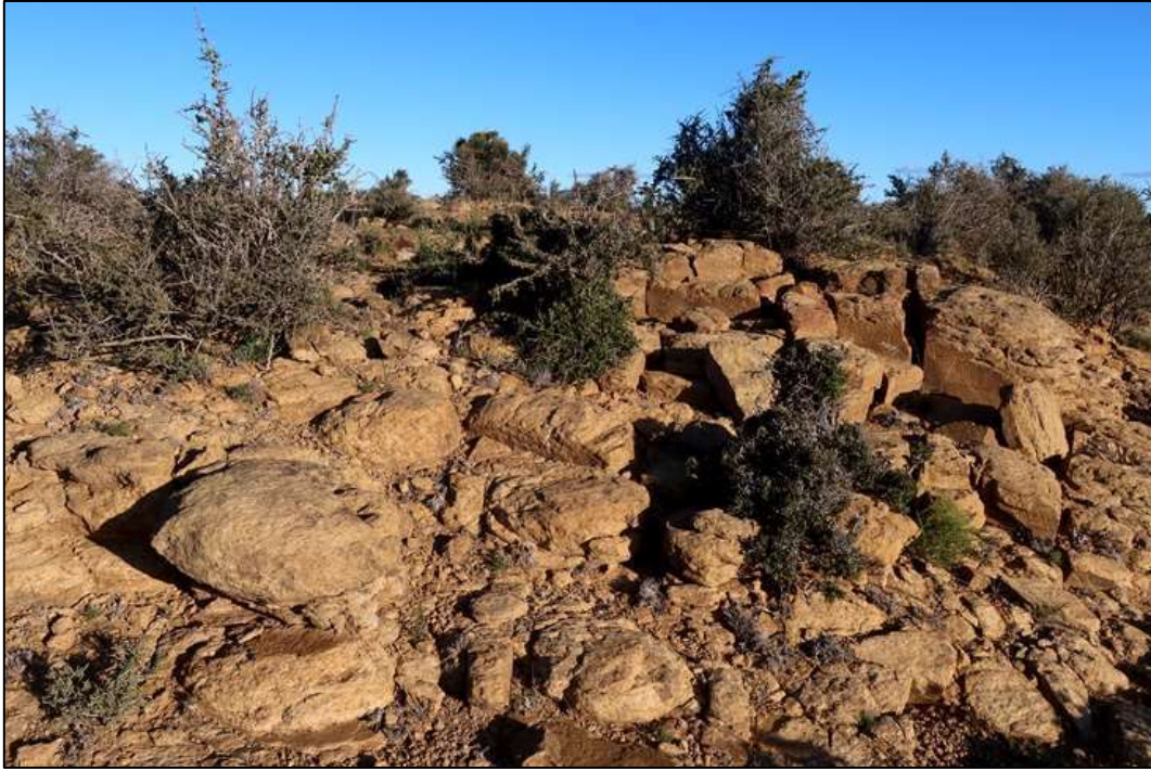
Figure 15: Distinctive, yellow-weathering, speckled, medium-grained channel sandstone facies building low ridges on Farm 94. This facies occurs commonly within the upper Abrahamskraal Formation and overlying Poortjie Member of the Teekloof Formation.
