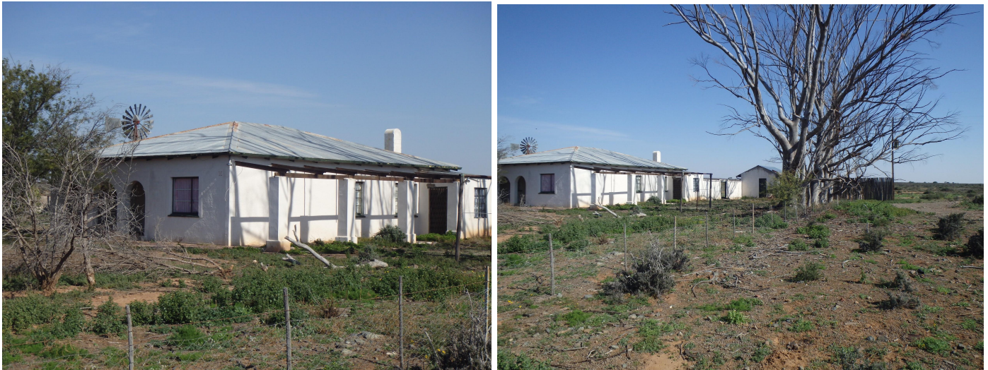
Figure 5.3: Observation ABD093 - Plaas 94, farmhouse complex, hipped corrugated iron roof, outbuildings
