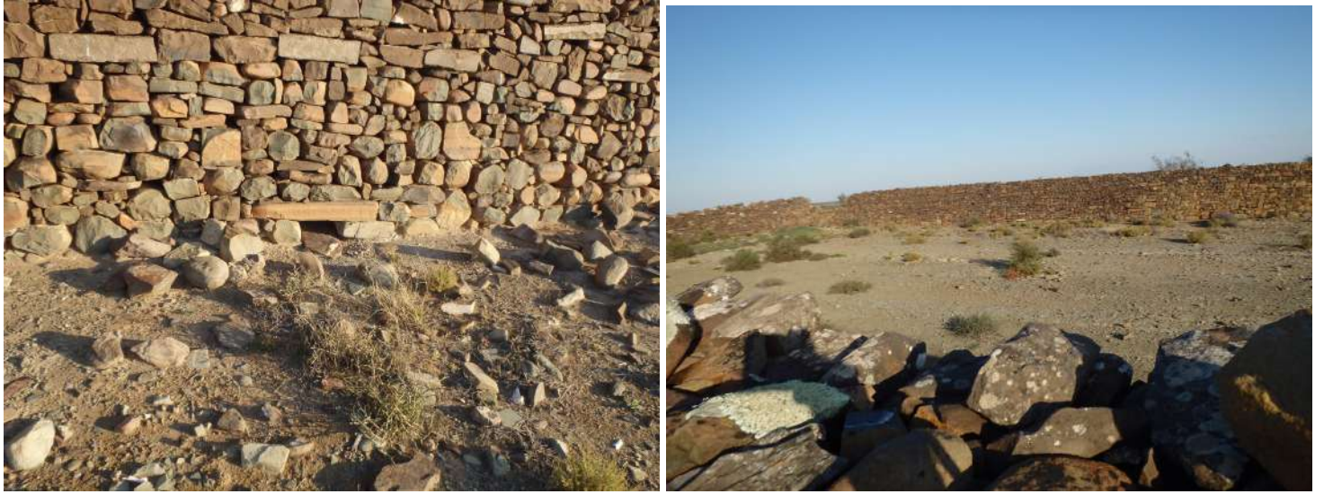
Figure 6.30: Observation ABD173 - Large vernacular stone walled kraal with high walls (2.5m high), local stone used and prominent marker on the landscape
