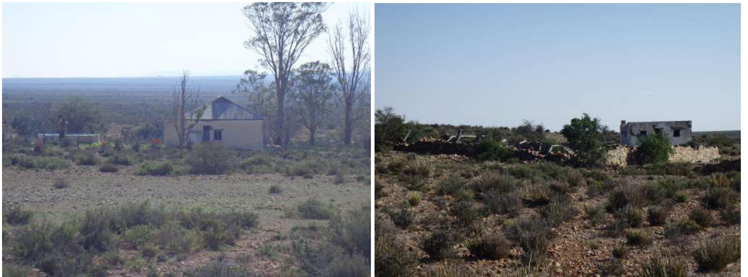
Figure 6.25: Observation ABD134 - Skoongesig farmhouse complex, kraals, Victorian hipped roof, corrugated iron
