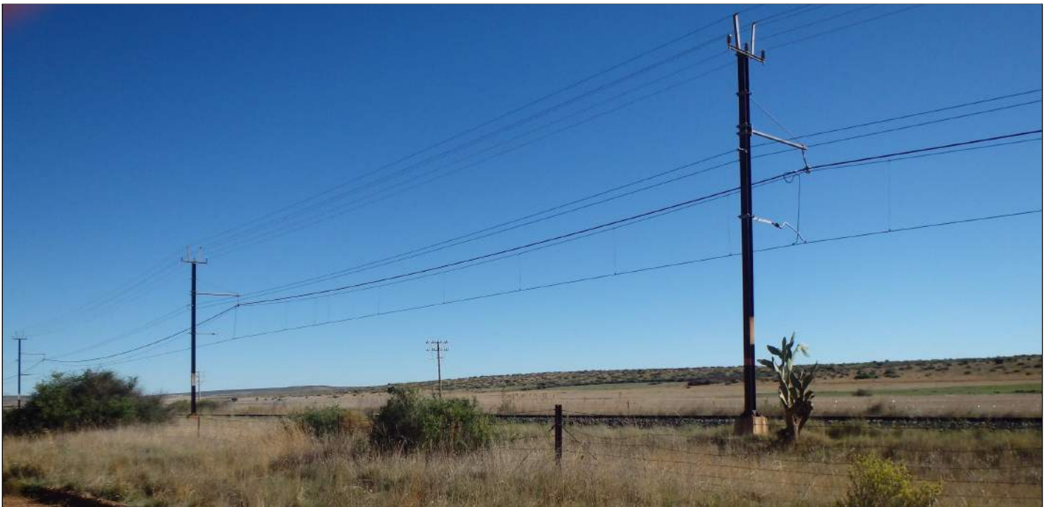
Figure 4.9: Contextual Images of Development Area indicating rail and electrical infrastructure
