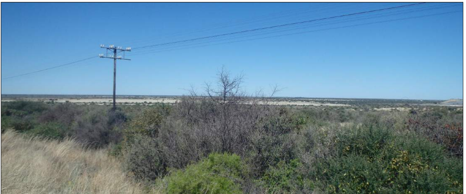
Figure 4.3: Contextual Image of development area indicating existing electrical infrastructure
