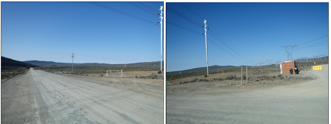
Figure 4.9: Contextual Images taken from the alignment running north-west to south-east indicating existing powerline infrastructure
