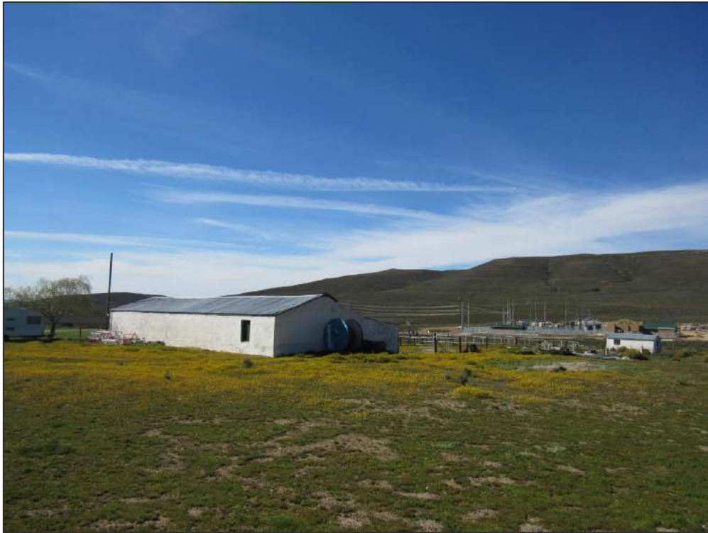
Figure 22: Bon Espirange Substation.
