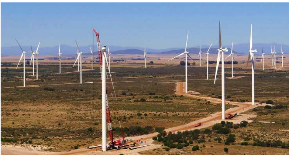
Figure 18. Wind farm and road infrastructure in the landscape: example of Wind Farm Hopefield with 37 turbines with a hub height of 95m and rotor diameter of 100m (total height 145m). (Image: Windbase.eu)
