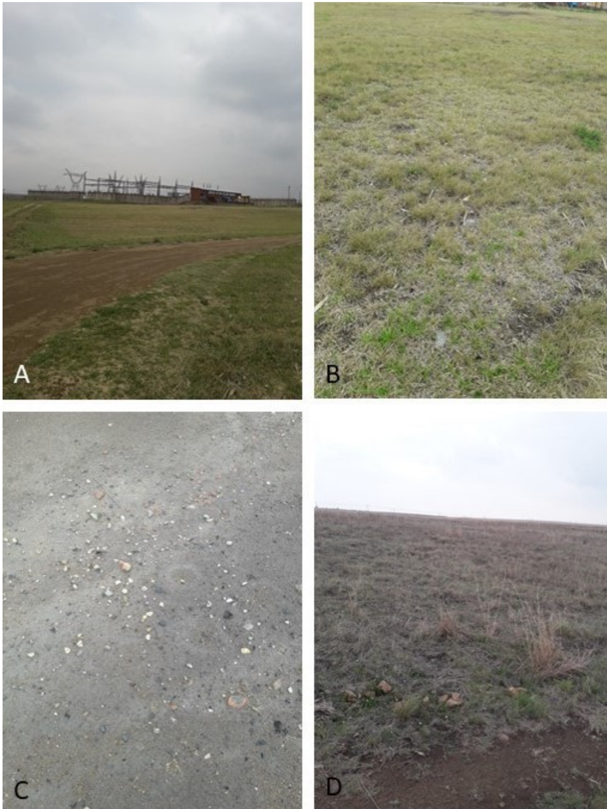
Figure 8: Photographs from the site visit to Goedehoop 290 IS Secunda PV facility. A-B = Stop 11, southern section of Betcrux 1 looking towards the existing substation on dolerite. C-D = Betacrux 3 (western project area). Stop 13. Gravelly soils but no rocky outcrops, and short grasses in most of the area. Disturbed area and no rocky outcrops or fossils were seen.
