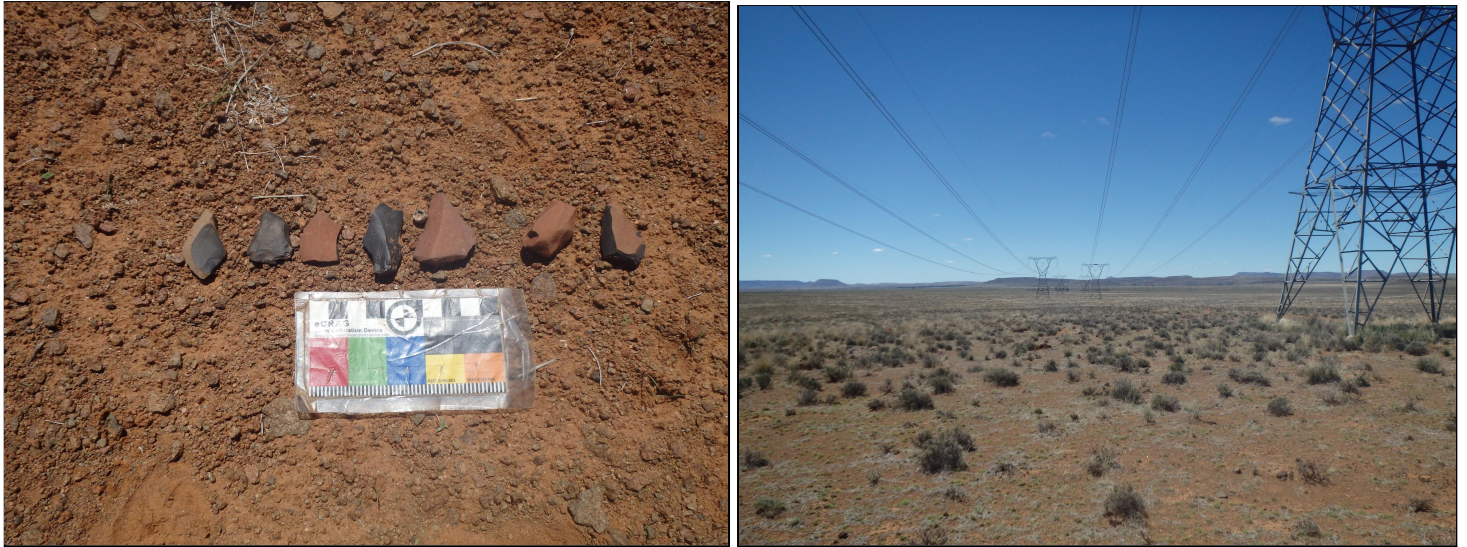
Figure 7.4: Observation Vetlaagte 032 adjacent to existing electrical infrastructure
