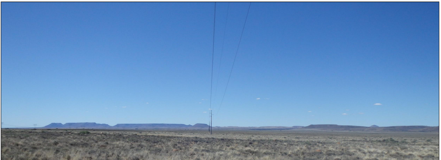
Figure 4.4: Contextual Images with existing electrical infrastructure
