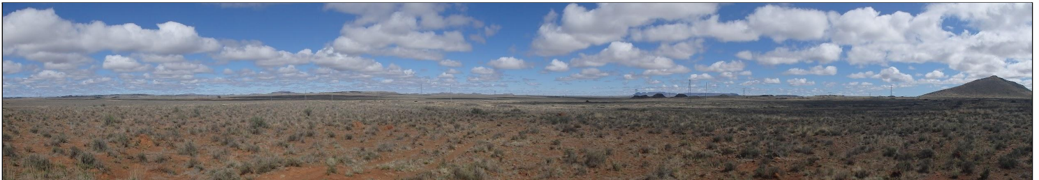
Figure 4.2: Contextual Images with existing electrical infrastructure
