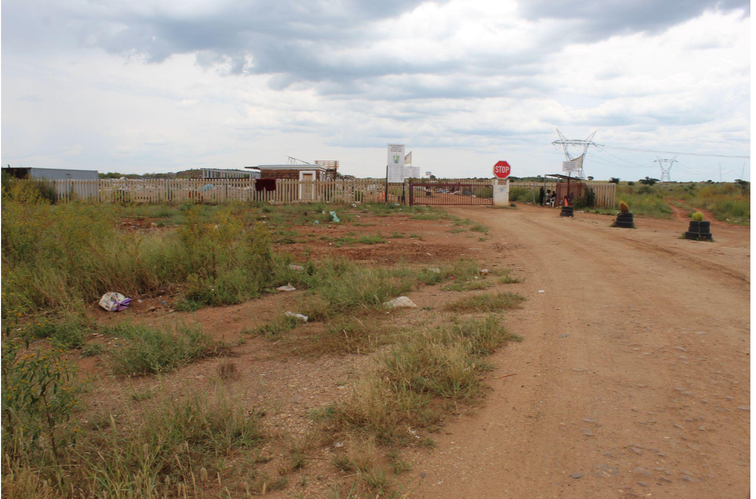
Figure 4.10 Contextual Images - Substation
