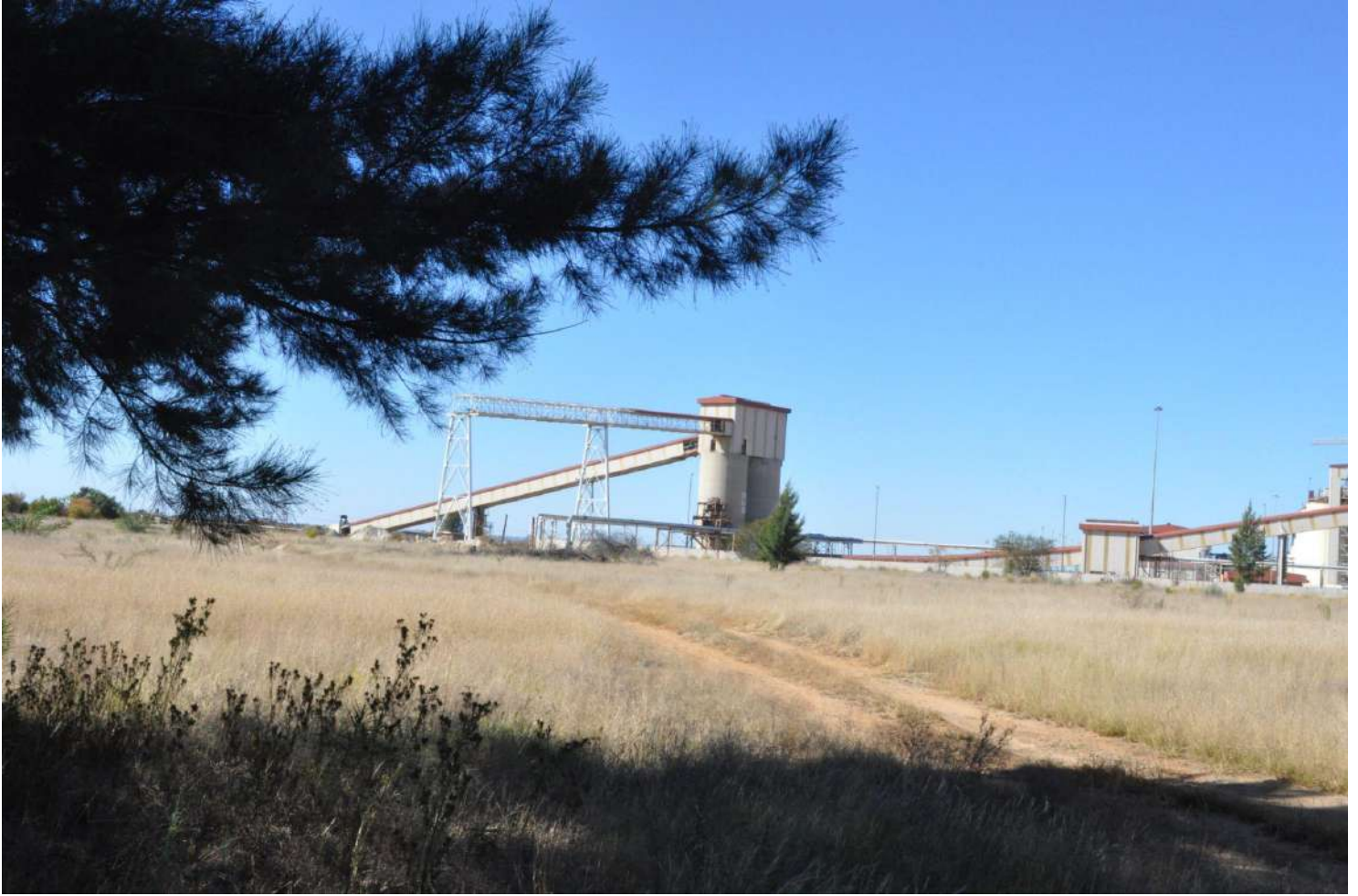
Figure 4.10: Areas of Central affected by mining activities: CCT1.
