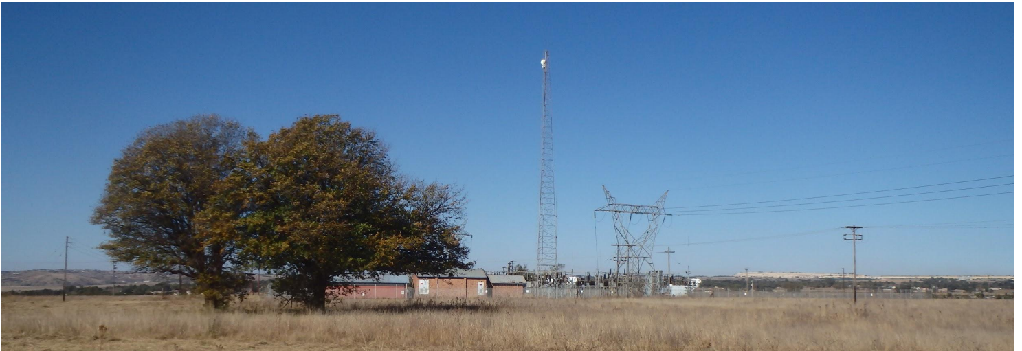
Figure 6.4: Observation 004 - Tarlton Substation
