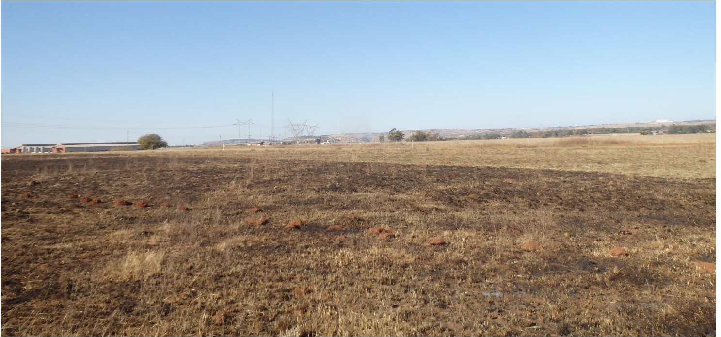
Figure 4.6: View of Tarlton substation and the Quantum factories to the left.
