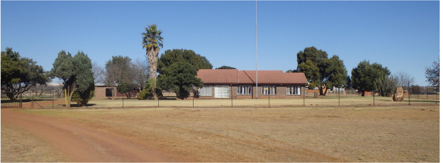
Figure 6.3: Observation 003 - Wolfelea Residence
