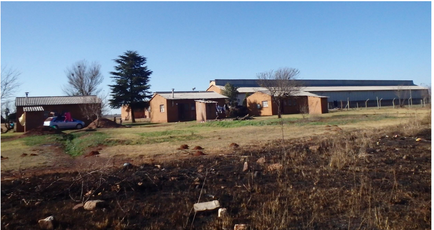
Figure 4.8: View of some of the staff buildings and chicken factory production facilities in the southern end.
