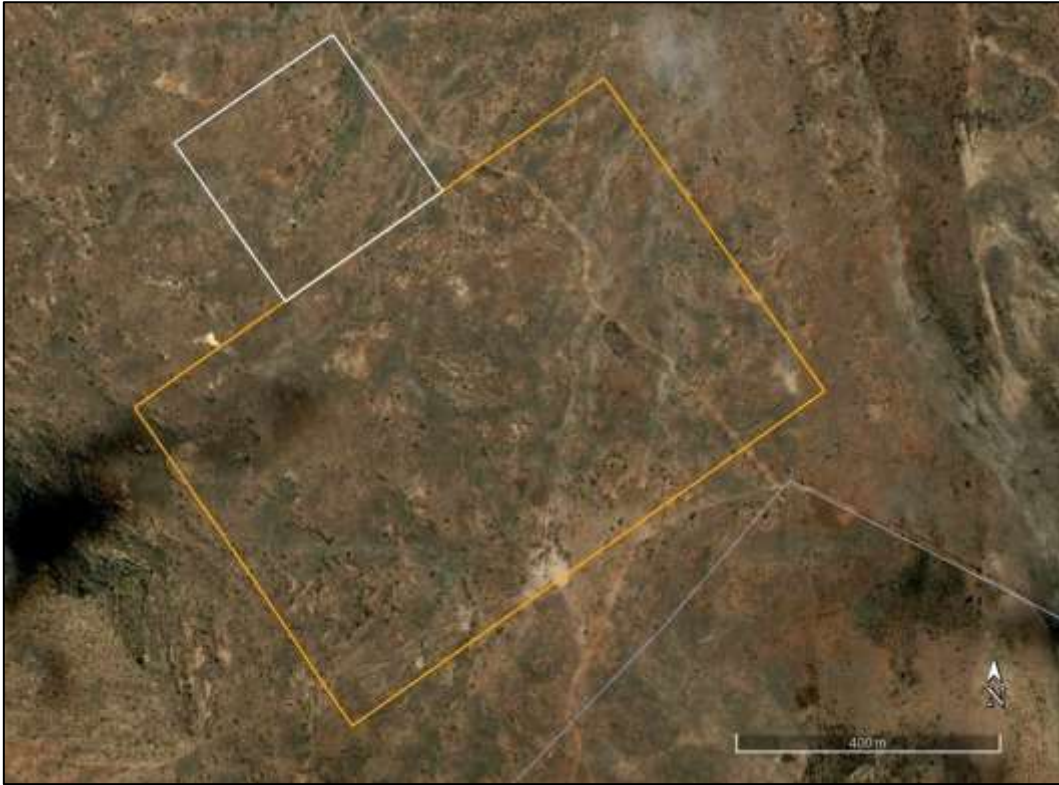
Figure 2: Google Earth© satellite image of the adjoining southern project areas situated on Portion 8 of Uitzicht Farm 3 and the RE of Elands Kloof Farm 135 (orange rectangle – substations, O&M buildings, overhead powerline; white square – CTMF).
