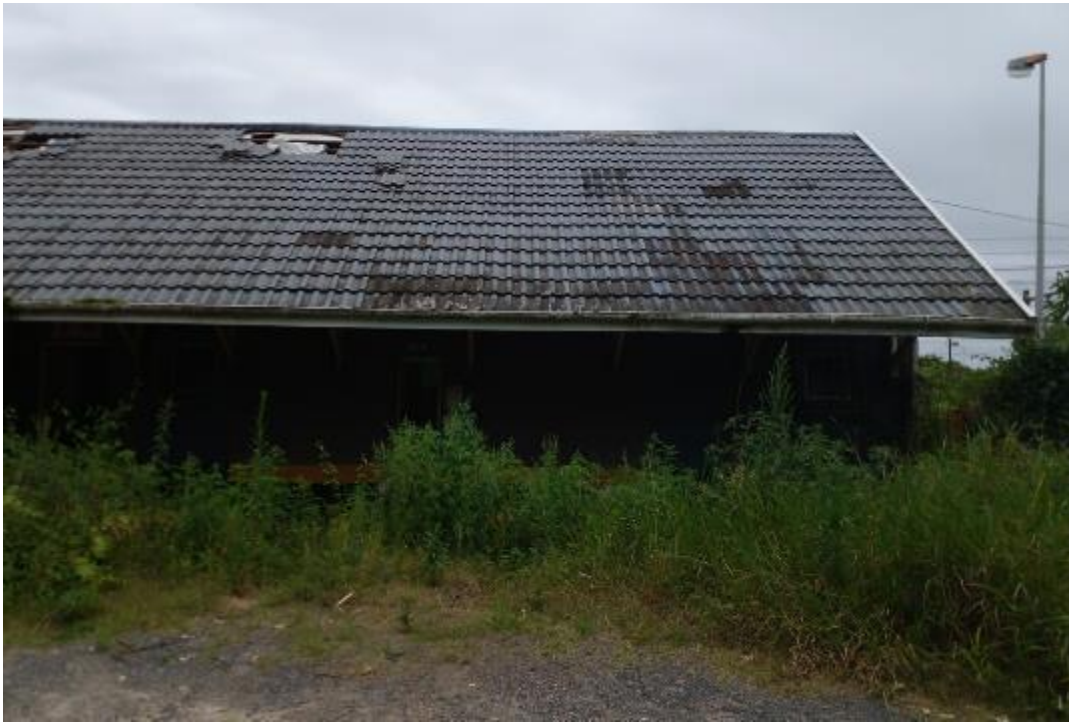
Figure 10: External view of section of railway station
