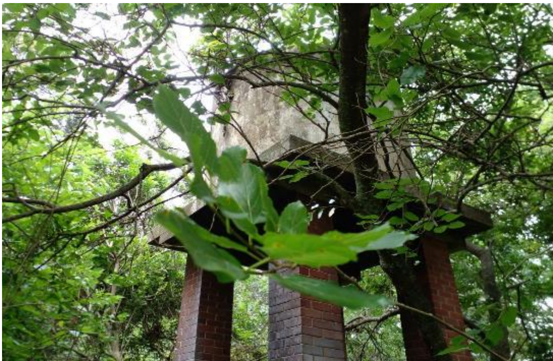
Figure 13: Elevated water tank on platform
