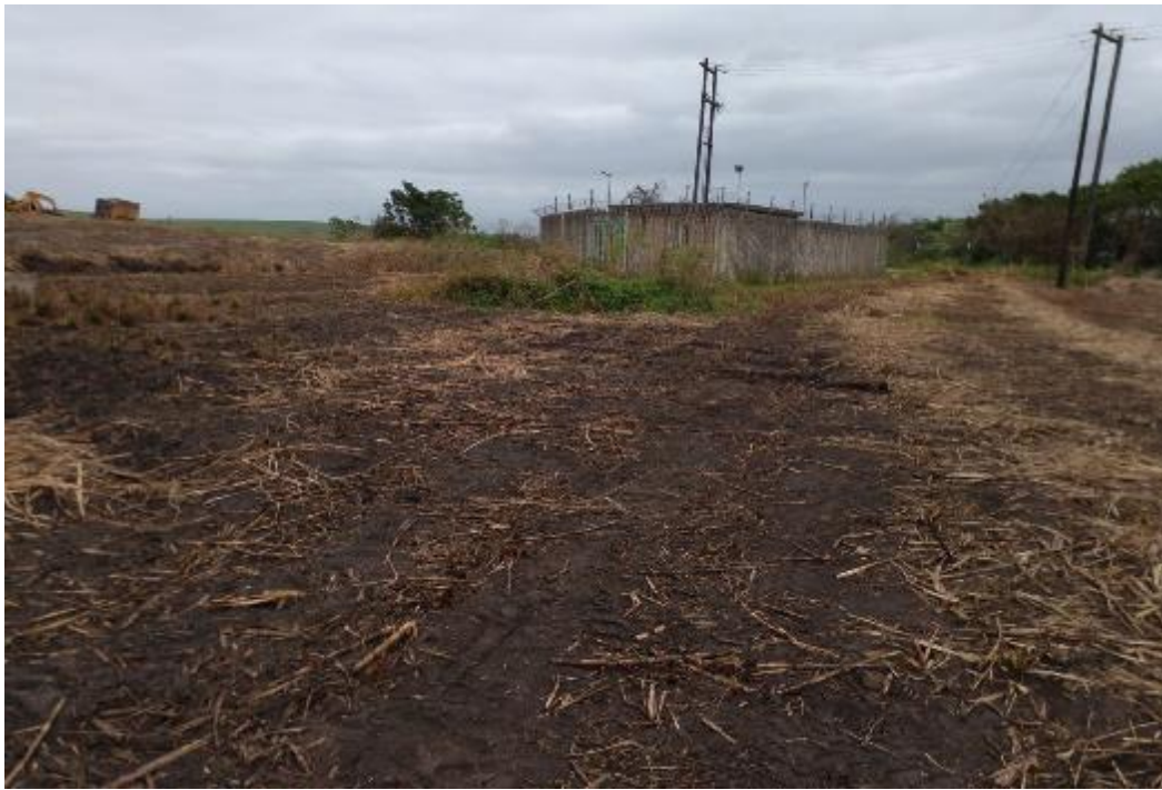
Figure 16: Compensation pump station
