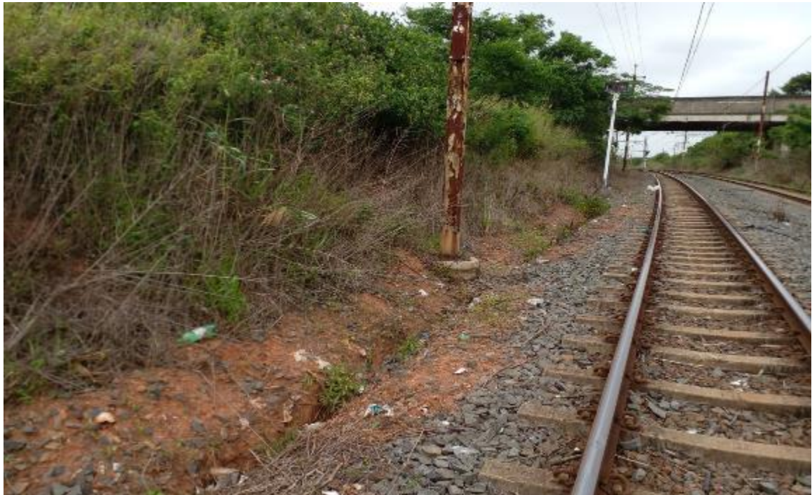
Figure 6: Pipeline route is situated close to railway line
