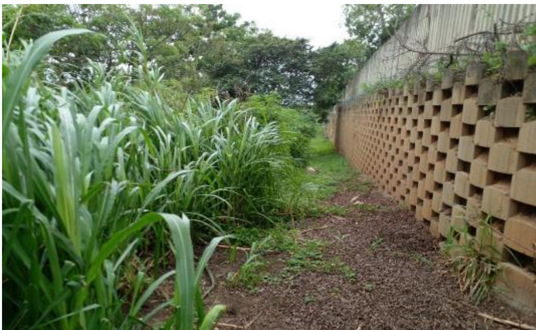
Figure 5: Pipeline route west of Estate boundary wall
