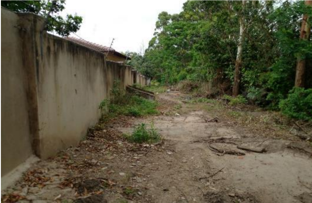
Figure 8: Boundary wall of Country Club and adjacent area
