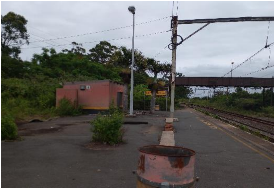
Figure 12: Railway line, platform and associated building
