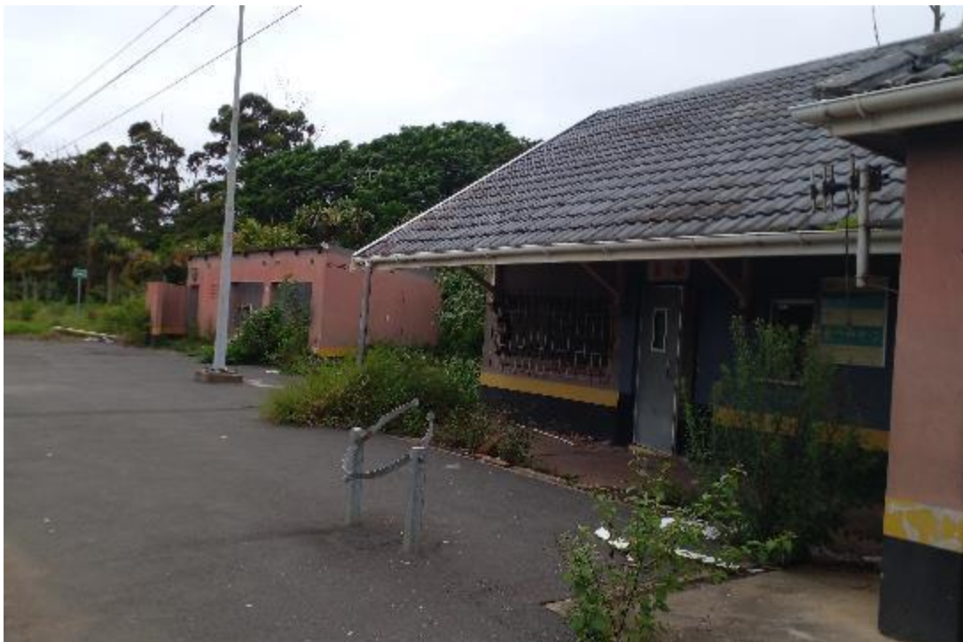
Figure 11: View of buildings and platform
