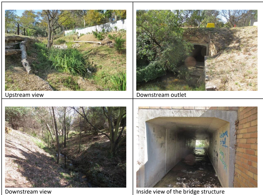
Figure 10. General views of the bridge structure
