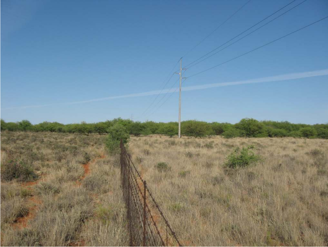
Photo 1: View of the power lines on the northern boundary of the study area.
