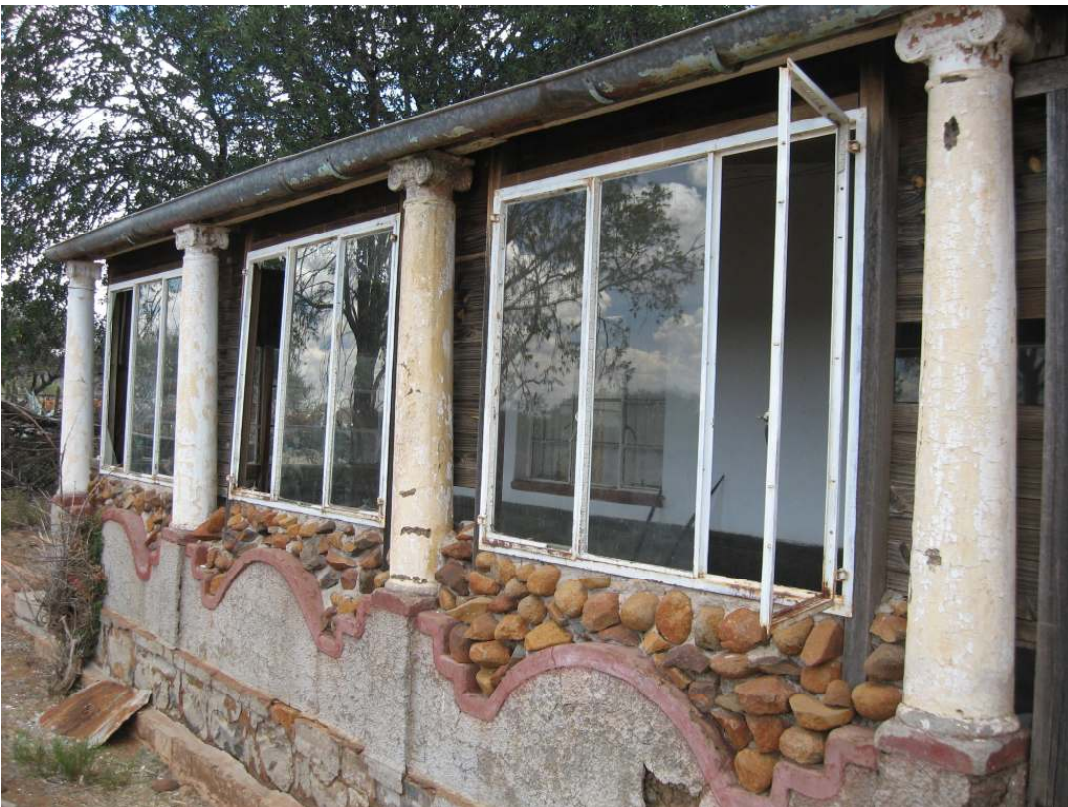
Photo 8: View of the closed up veranda as a later addition.
