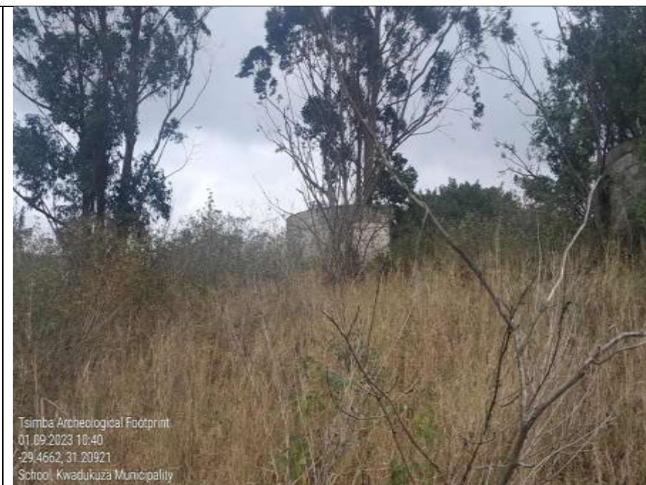
Figure 4: View of an abandoned structure with trees growing inside
