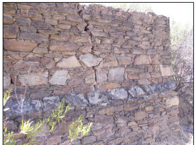
Figure 26: The southern wall of the added on room.
