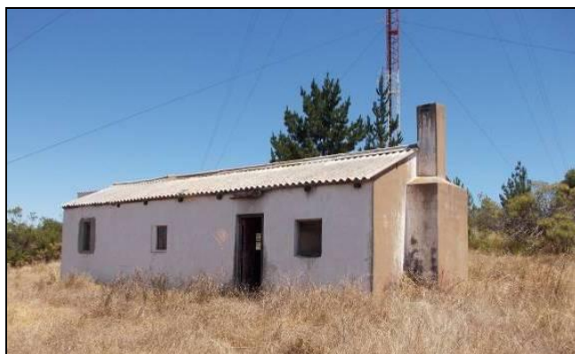
Figure 39: Mid-20 th century cottage at point 008b. It has an asbestos roof.
