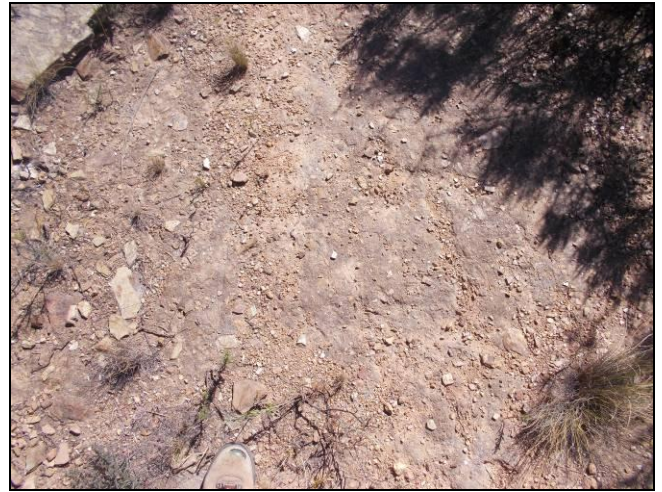
Figure 24: The road surface on the 1899 pass.
