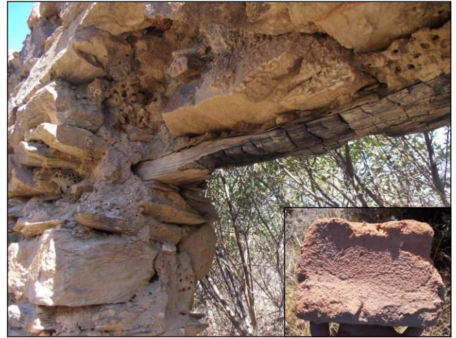
Figure 28: Detail of window in north-western part of the house.
