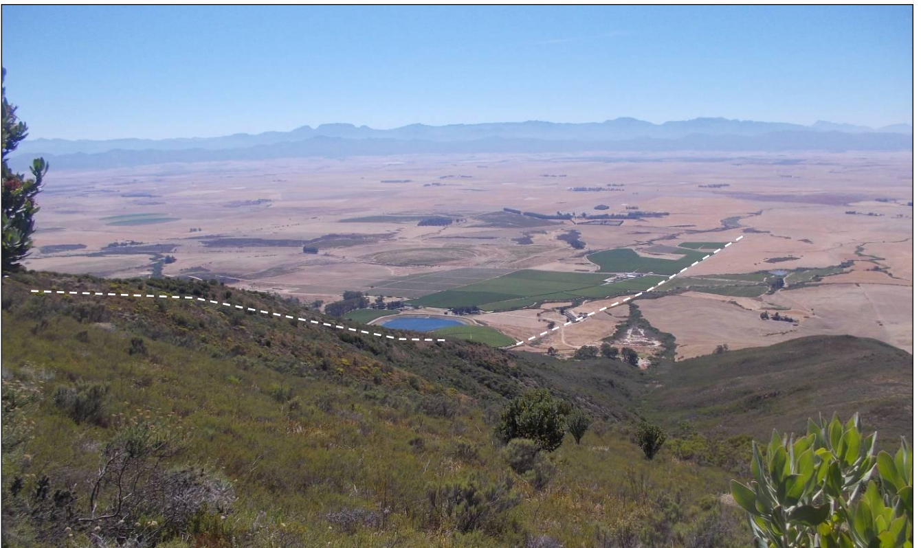
Figure 9: View east from the top of the mountain showing the alignment of Alt. 6 (white dashed line). It turns leftwards (northwards) off the ridge before running past the vineyards at the foot of the mountain.
