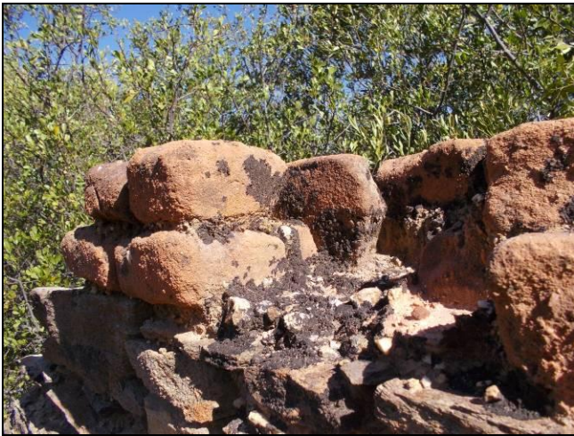
Figure 27: detail of bricks atop the stone walling on the north-western part of the house.
