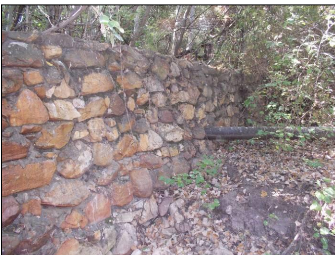
Figure 30: The dam wall at KV2013/002 (point 010).
