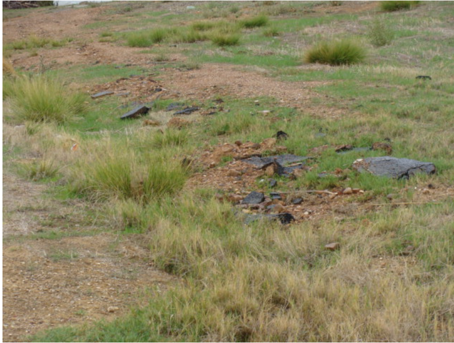
Figure 11 Compacted material in the surveyed area.
