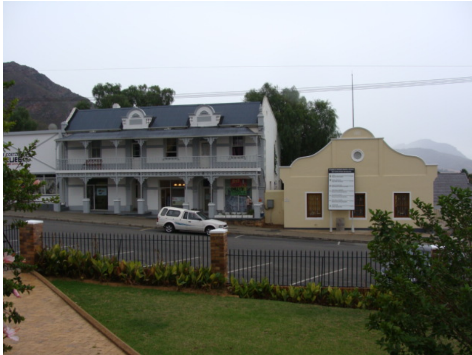
Figure 15 Late 19 th / early 20 th century historical buildings in Piketberg.
