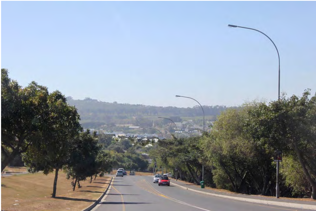
1B: Simulation: view approaching via Jip de Jager Drive - tree planting to provide screening.
