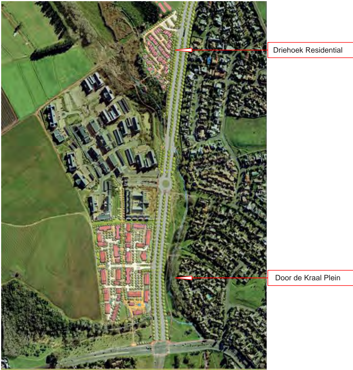
Driehoek Residential, Door de Kraal Plein and Jip de Jager extension in context (Image source: OVP Associates)
