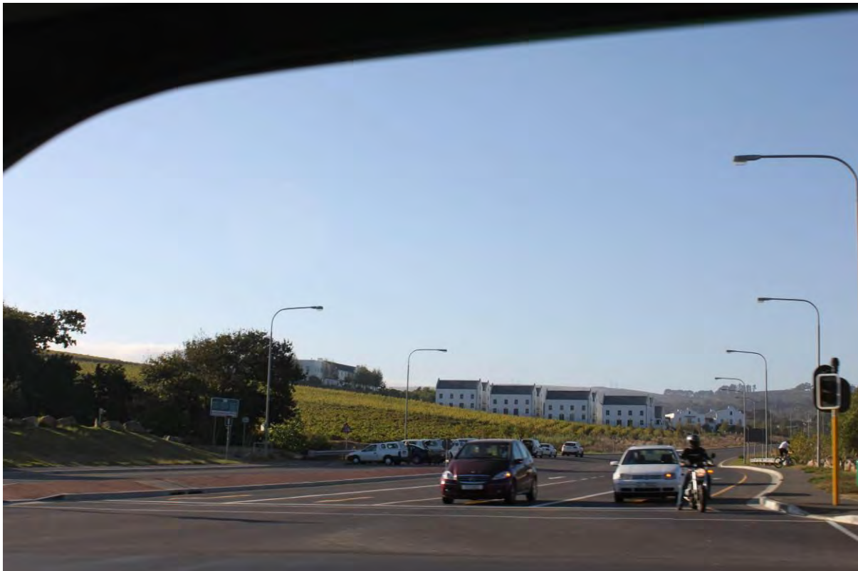
33: Intersection of Van Riebeeckshof Road and Jip de Jager Drive looking northwards - refer to photomontages 33A (un-mitigated) and 33B (mitigated)
