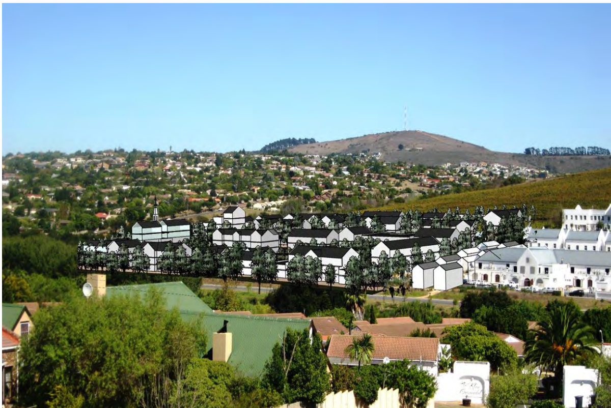
Additional Image: Source: Boogertman and Partners. (Based on these, the decision was taken to reduce the 6-storey block by one storey)
