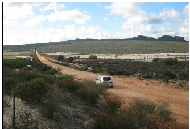
Figure 12: View north showing sand in road reserve. Note also the disturbed strip along the east side of the road.
