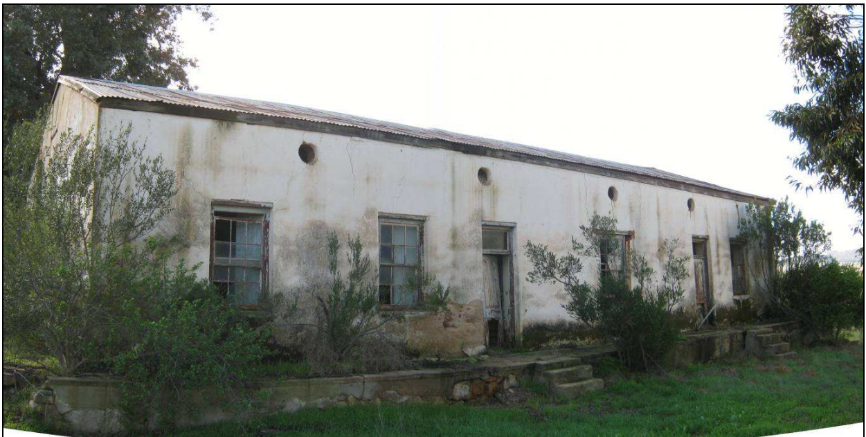
Figure 14: View of the front of the 19 th century house.
