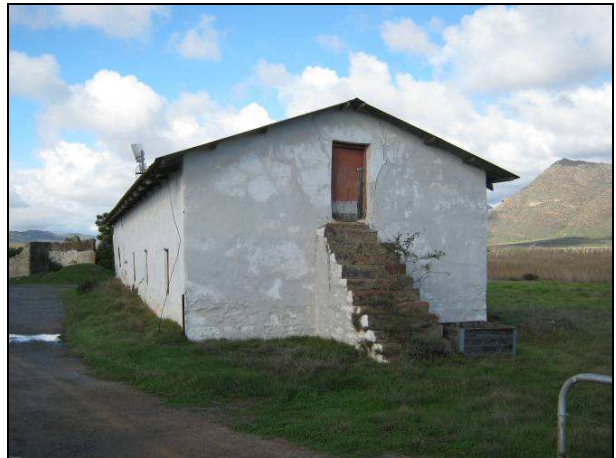
Figure 18: View of the west end of the 19 th century barn.
