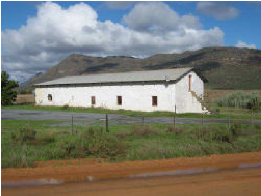
Figure 15: View of the 19th century barn east of the (ACO 2011: 11)
