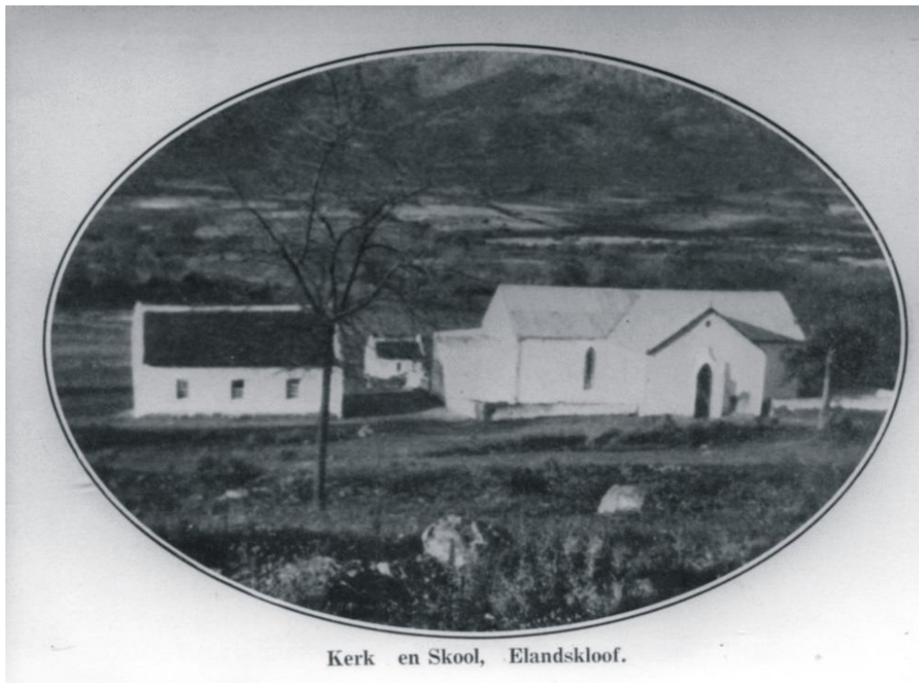
Figure 12: Church and school in 1932. At that time the school must have been a single classroom and the porch to the church had yet to be built. Note the current holbol gable was also not then in existence and there appears to be a lean-to addition at the north end
