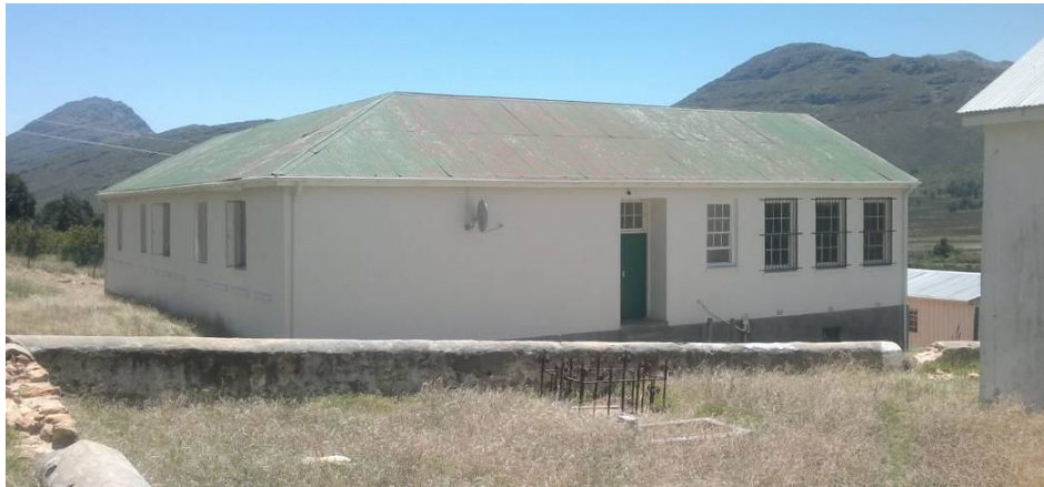
Figure 21: The school is sited close to the northwest of the church enclosure
