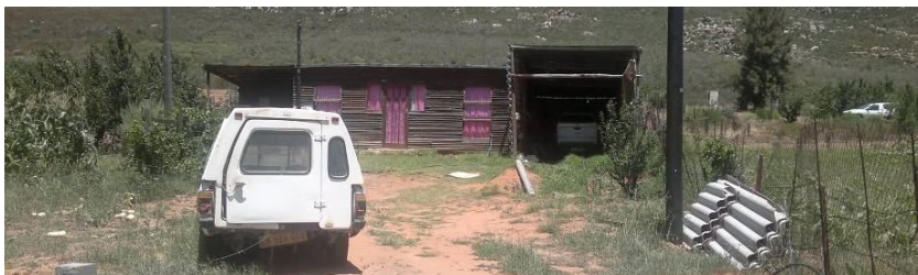
Figure 27: Small timber frame structure
