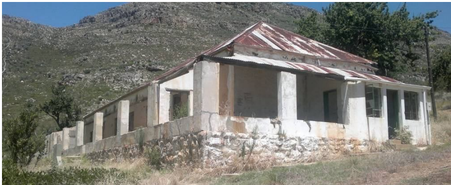
Figure 19: A veranda once ran along the entire front façade and around each end. The stoepkamer on the right functioned as an office
