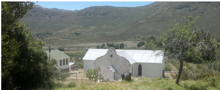
Figure 14: The main entrance to the church is from a small porch but there are also doors at each gable end. The school is on the left
