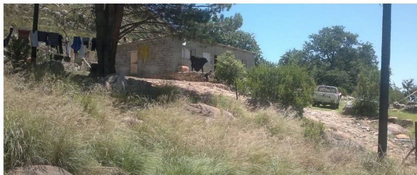
Figure 25: Masonry structure that appears to have been built on the original cottage platform
