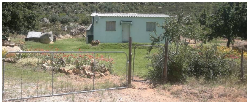
Figure 26: Small dwelling of masonry construction built on the original cottage platform
