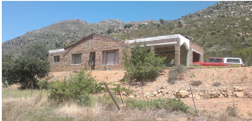
Figure 24: Substantial house built recently on a terrace site at the south west end of the valley. As can be seen a seen there has been considerable cut and fill creating an unsightly bank of exposed rubble
