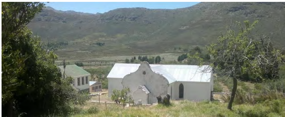
Figure 14: The main entrance to the church is from a small porch but there are also doors at each gable end. The school is on the left
