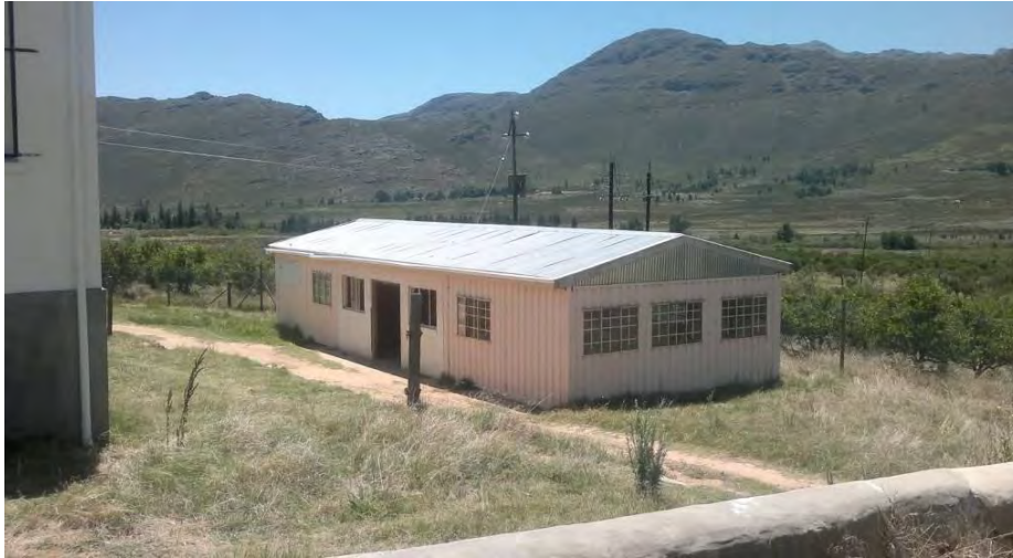
Figure 33: Steel framed pack shed close to the citrus orchards
