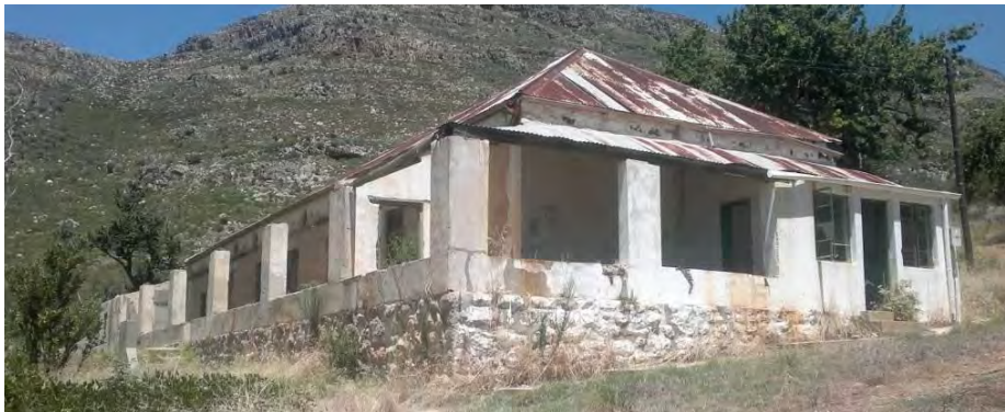
Figure 19: A veranda once ran along the entire front façade and around each end. The stoepkamer on the right functioned as an office
