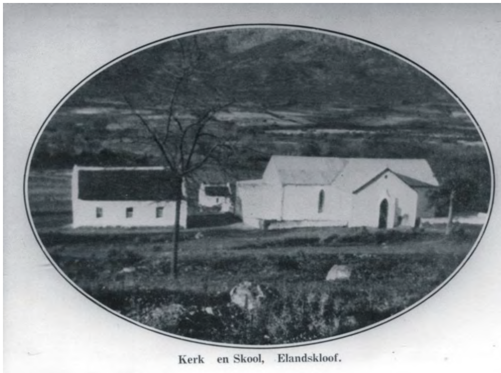
Figure 12: Church and school in 1932. At that time the school must have been a single classroom and the porch to the church had yet to be built. Note the current holbol gable was also not then in existence and there appears to be a lean-to addition at the north end
