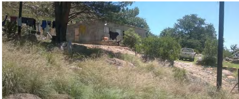
Figure 25: Masonry structure that appears to have been built on the original cottage platform
