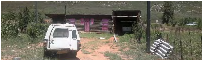
Figure 27: Small timber frame structure
