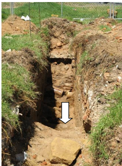
Figure 44: Test Trench A: the arrow shows the position of the streambed, and the position of the test into the cobble bed (Photo taken facing west/southwest).
