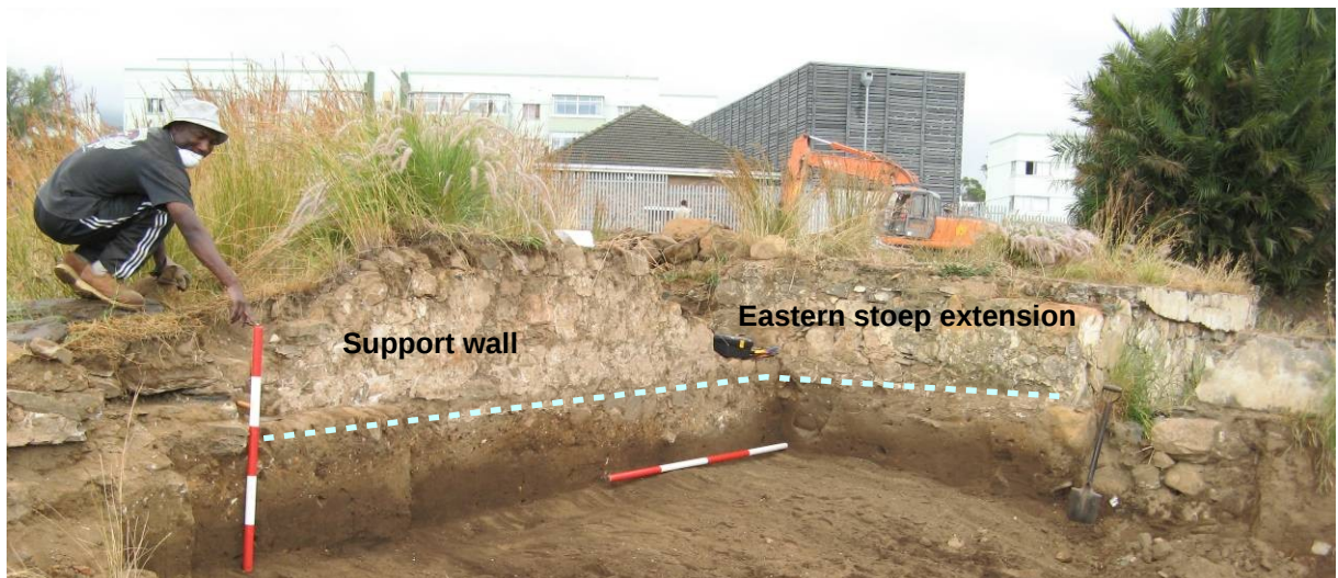
Figure 21: The blue dotted line shows the level of the mid 19 th century ground surface. This level is confirmed by the remains of a cobble layer (just to the west of the 1m measuring rod) and the extent of the plaster mark. The slate pavers shown in Plate 14 were also located at this level.
