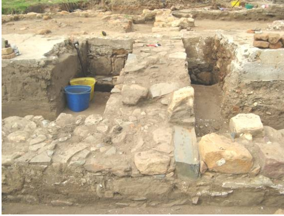
Figure 7: The construction method used in the stoeep is similar to that used in the original core, but with a brown clay mortar. NW corner.
