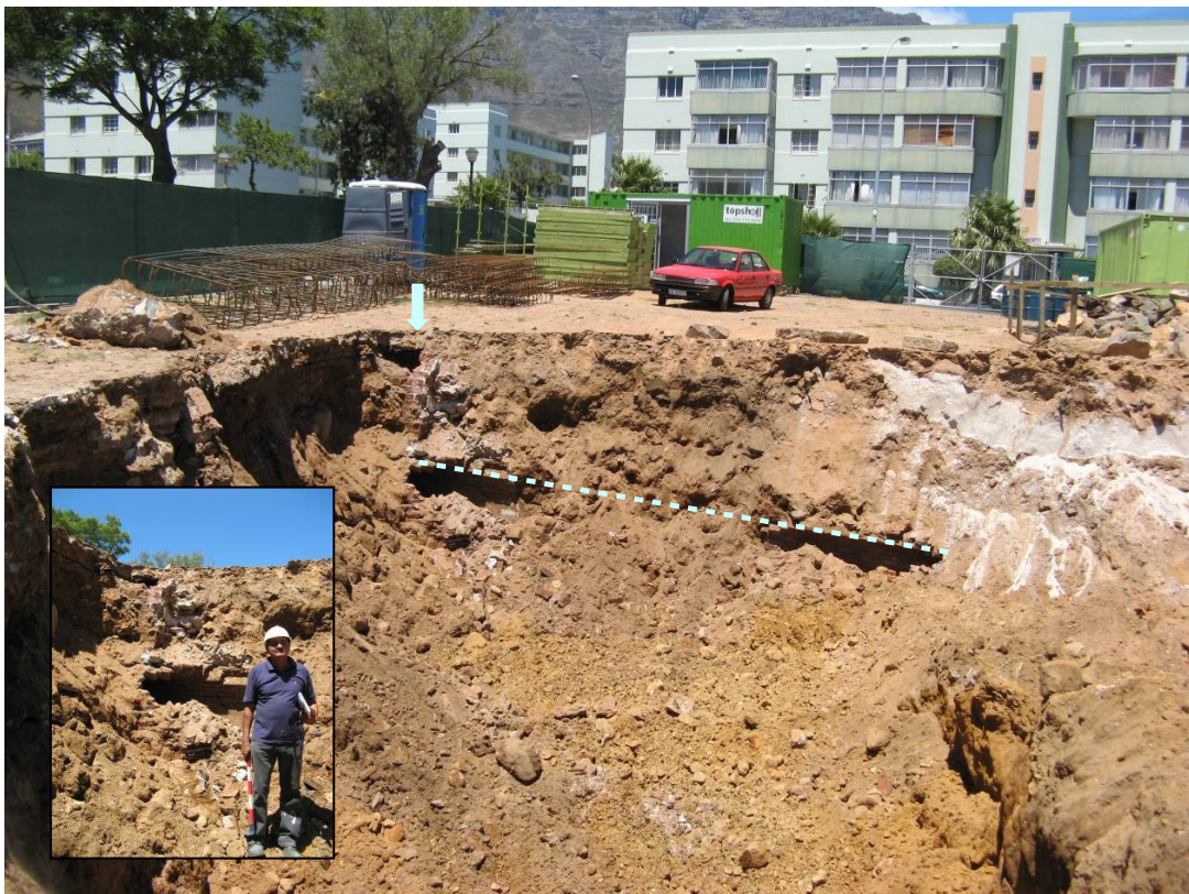
Figure 52: Location of the drain on the southern side of the substation. Top of the drain is highlighted by dashed line. The arrow shows the location of a stop point in the line (Detail shown on insert and Figures 53 and 54).
