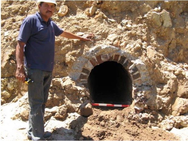
Figures 50 and 51: Detail of the drain to the north of the substation. Image on the right showing detail of the interior of the drain.
