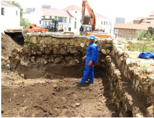
Figure 9: Views of Wall 4A. Note the similar construction method to the core. Varying depths of foundation is very clear in the image on the right. (Image on the left is taken facing N. Image on the right was taken facing SE).
