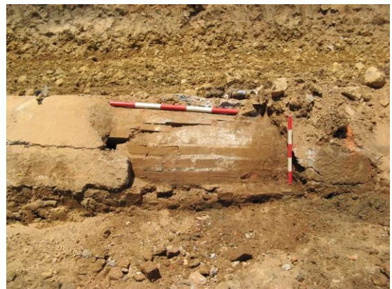
Figure 49: Detail of the drain to the north of the substation. 19th century brick with clay mortar, covered by a thick layer of coarse cement characterises the drain.
