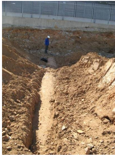
Figures 46 and 47: View of the uncovered drain to the north of the substation (Photos taken facing south). The drain sloped towards Mount Str: this section still containing water ).
