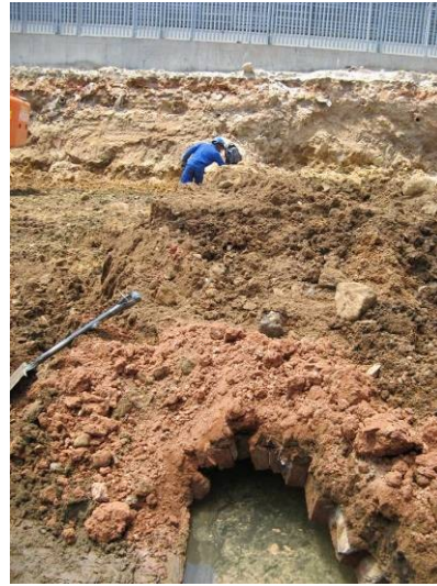
Figures 46 and 47: View of the uncovered drain to the north of the substation (Photos taken facing south). The drain sloped towards Mount Str: this section still containing water ).
