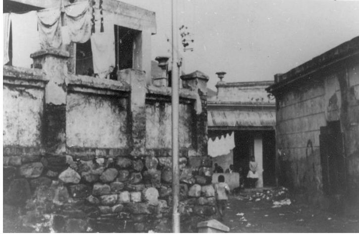
Figure 37: Oblique view of the NW corner of the Welgelegen dwelling. The stone walling of the Stoep Area II is shown with its brick and mortar walling. The building in the background is part of a row of semi-detached cottages facing onto a lane giving onto Mount Street. (Cape Archives AG17606).
