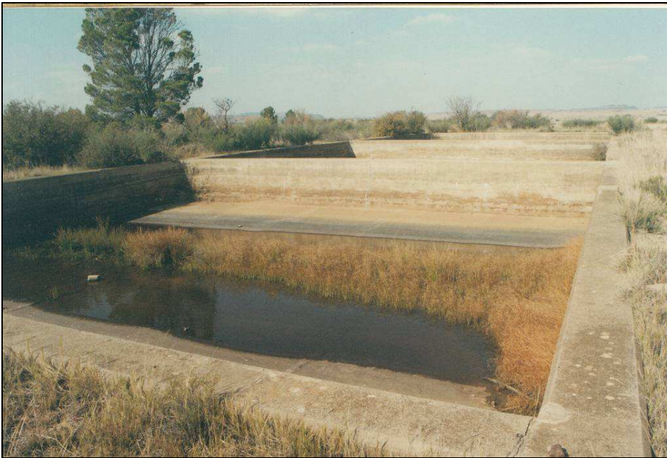
Fig.17 Old water reservoir dams at the Modder River pump station.
