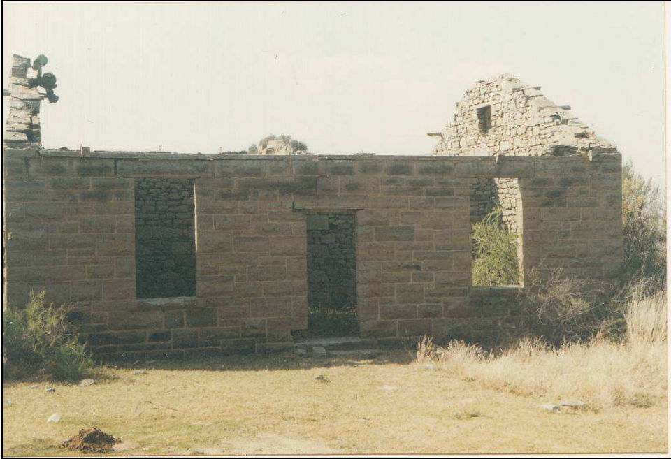
Fig.16 Sturdy old building at the Modder River pump station.
