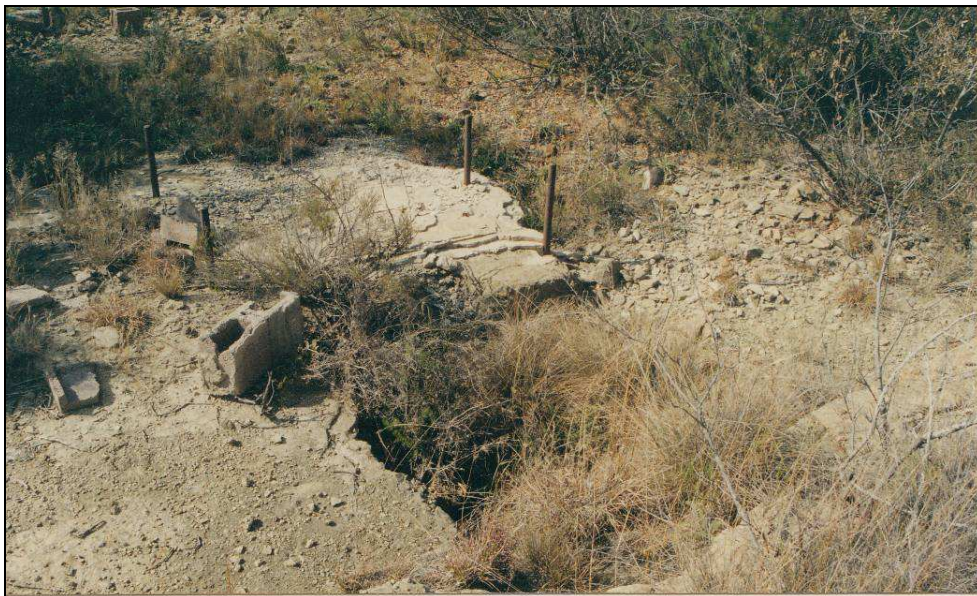
Fig.15 Fixtures for the steam engines in what used to be the pump house at Modder River.
