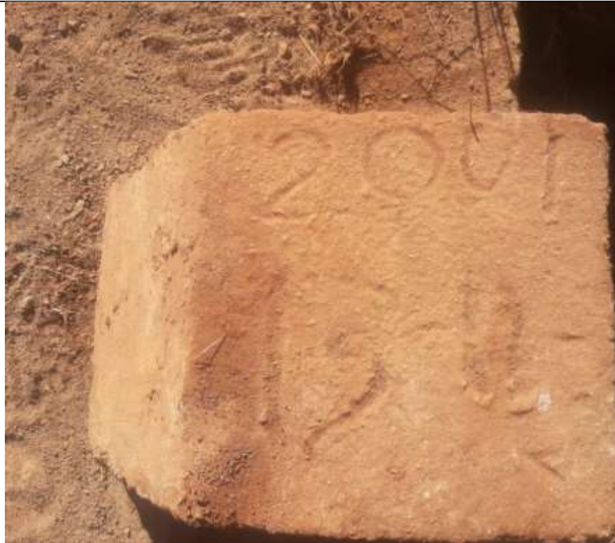
Figure 19: View of scribed concrete slab showing the year the bridge was built
