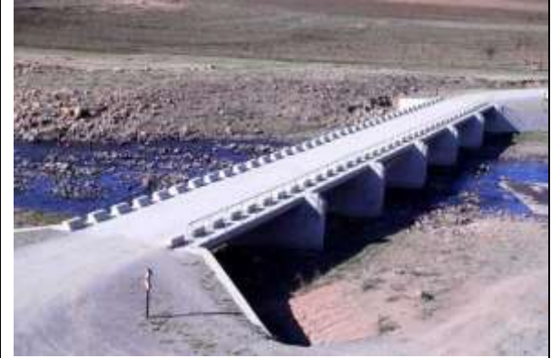
Figure 23: Gungununu River bridge (2018)
