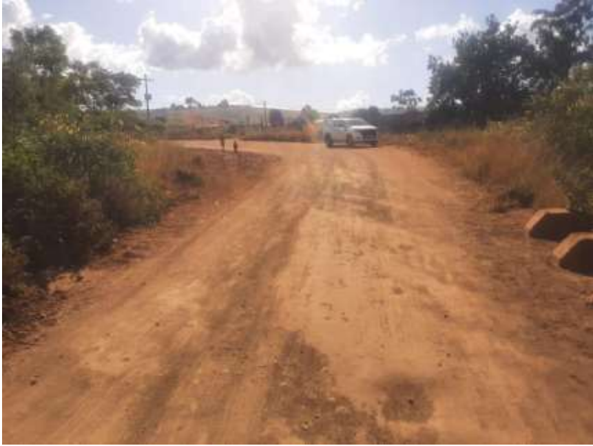
Figure 9: View of the bridge from the downward depression
