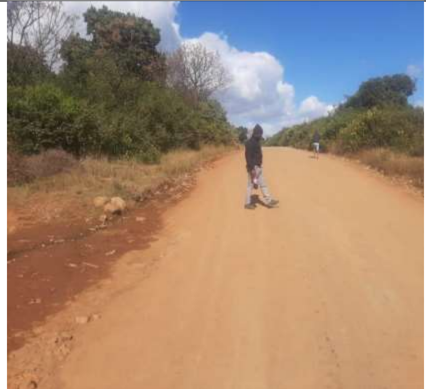
Figure 20: View of another area to be affected by the culvert
