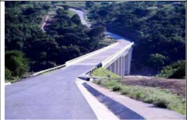
Figure 26: Nyakana river bridge (2018)
