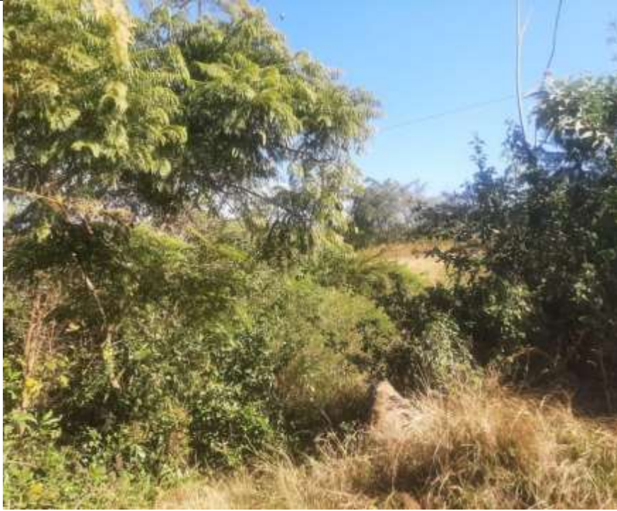
Figure 17: View of a water pipe covered in dense vegetation
