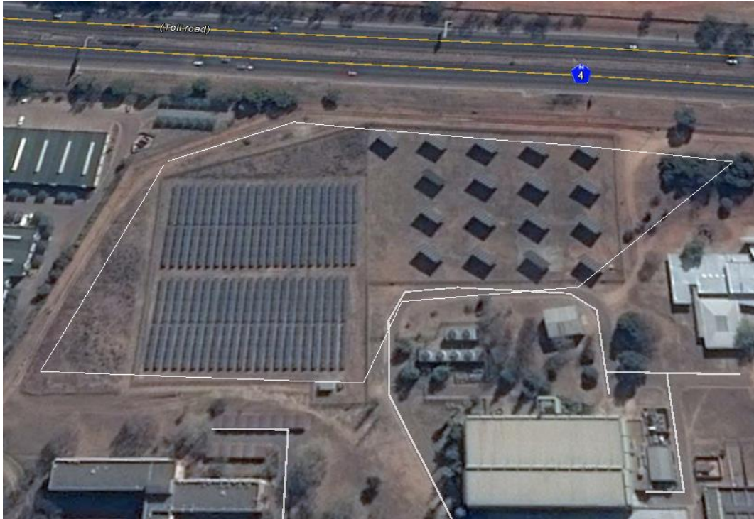
Fig 10. View of Site 3 adjacent to the photovoltaic plant.
