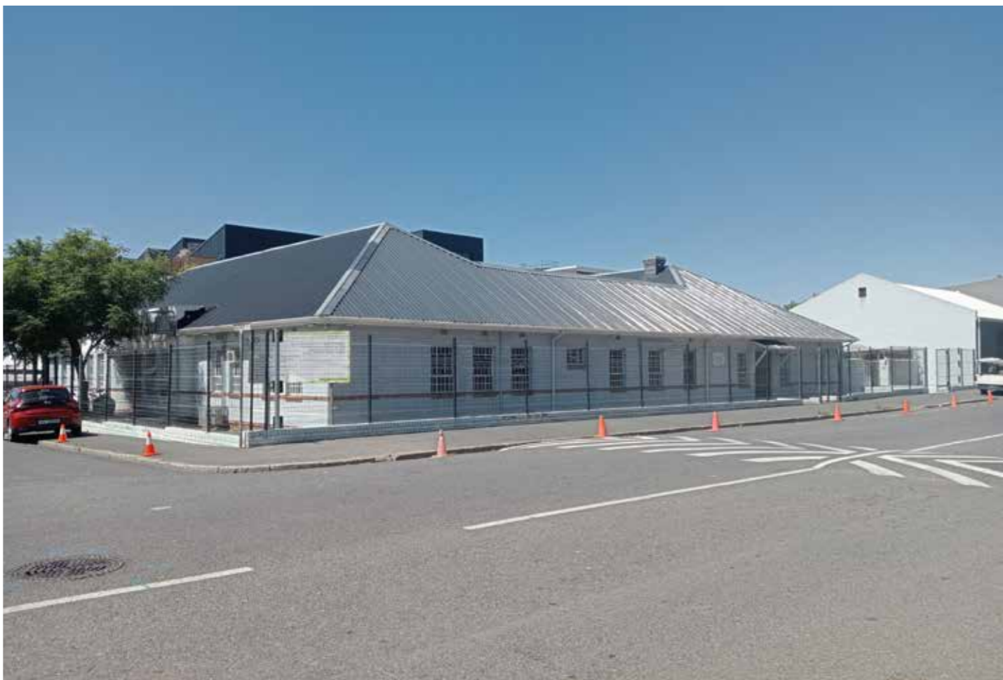
Figure 7. Woodstock Clinic, view to north east (RSA, 2022)
