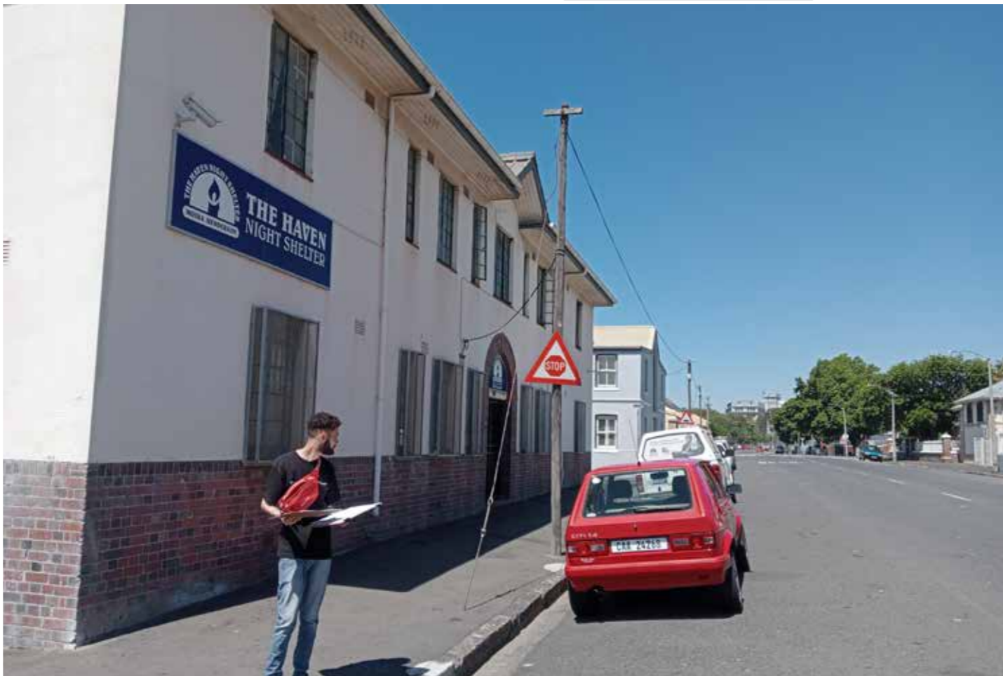
Figure 9. The Haven Night Shelter, view to south east (RSA, 2022).
