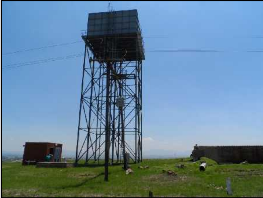
Figure 10- Example of Charlestown water works
