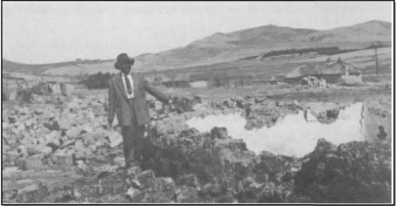
Figure 21 - A photo showing a man point to the ruins of his house following its demolition by the Nationalist Government in Charlestown to make way for white residents
