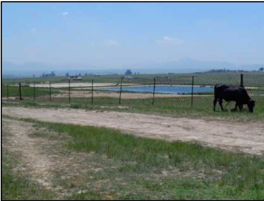
Figure 9—Example of Charlestown water works
