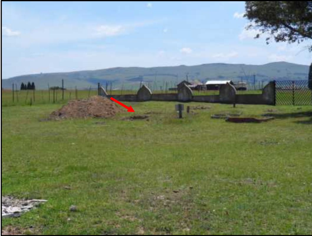
Figure 36 - Graves with the Mausoleum. Note the active grave-pits as indicated by the red arrow and the cement and brick dressing, as well as the cross headstone.
