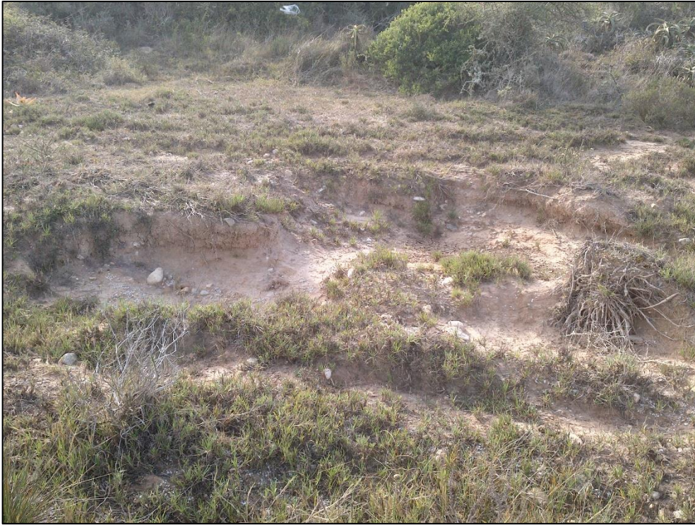
Figure 8. View of an exposed surface erosion area investigated.
