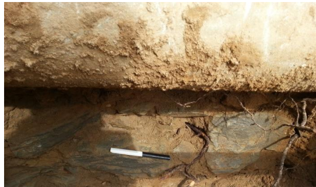
Figure 4 At the entrance to the pavement testing laboratory the foundations of a stone wall that ran across Chiapinni Street were encountered.
