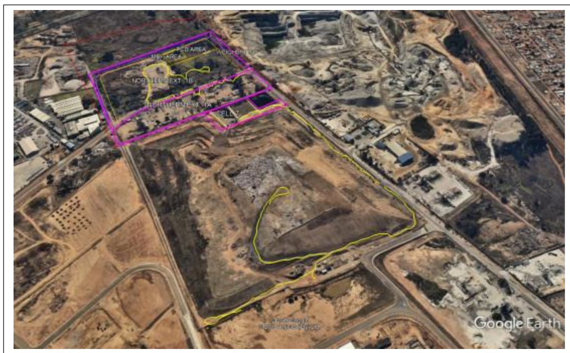
Figure 3- GPS track log which was registered with a mounted GPS instrument (yellow outline). Pedestrian surveys were conducted from the main pathway. Not all tracks were recorded (above).
