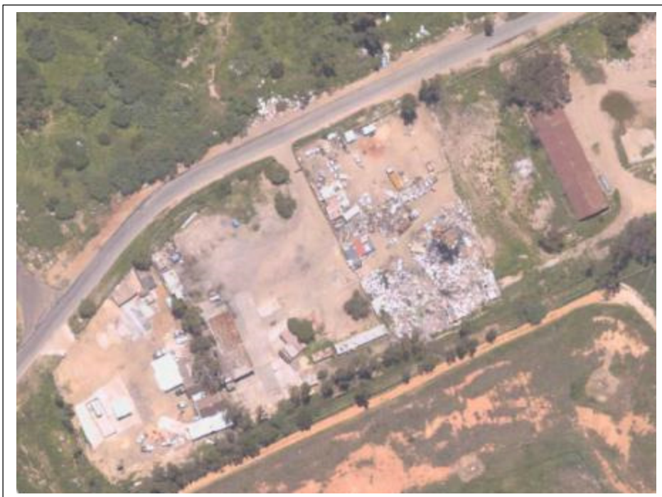
Figure 7– Northern Extension Area 1 A is used for various activities such as crushing, recycling of waste materials, dumping, etc. The workshops and other infrastructure in this area hold no heritage significance (above).
