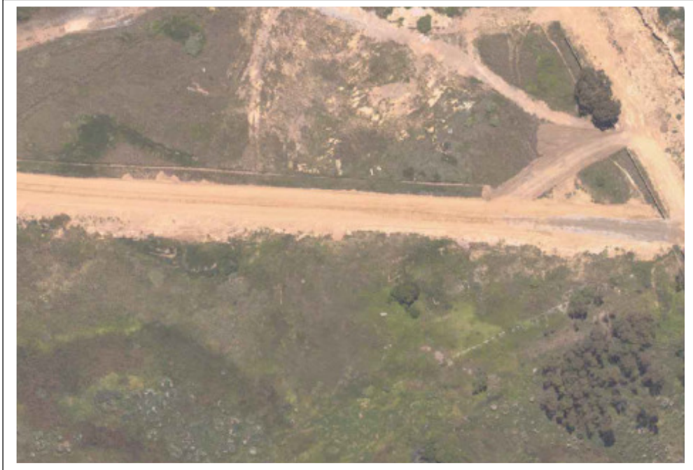
Figure 9- The northern part of Northern Extension Area 1 A where the PCD and MRF will be established has been scarred by road construction and the removal of soil and have left the area in a negative environmental state (above).
