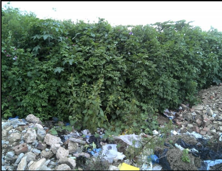
Figure 14. Shoulder high vegetation and dumping.
