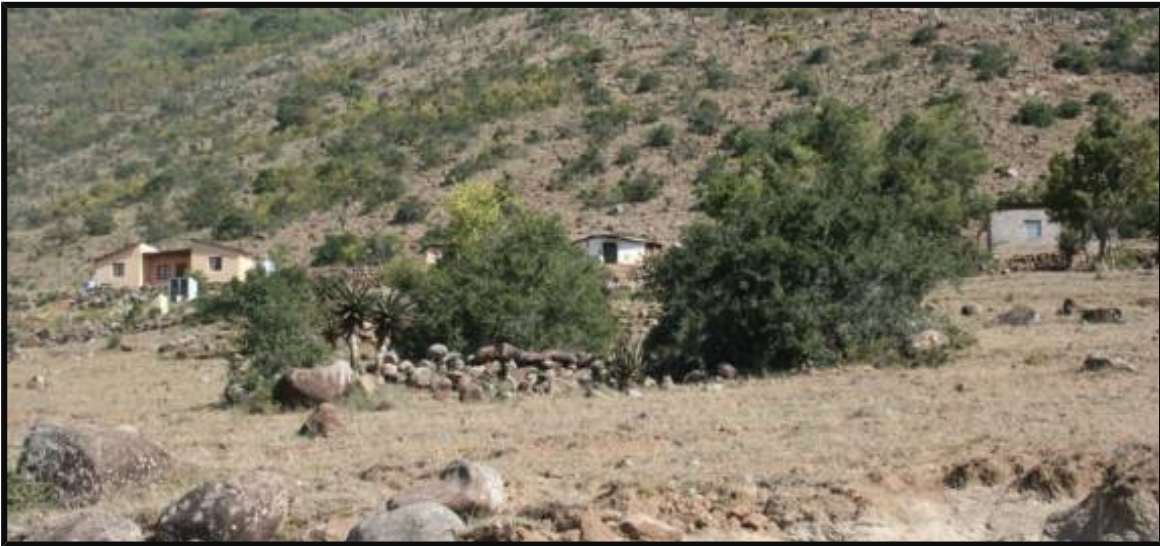
FIG. 7: STONE WALLING AT CHC09
