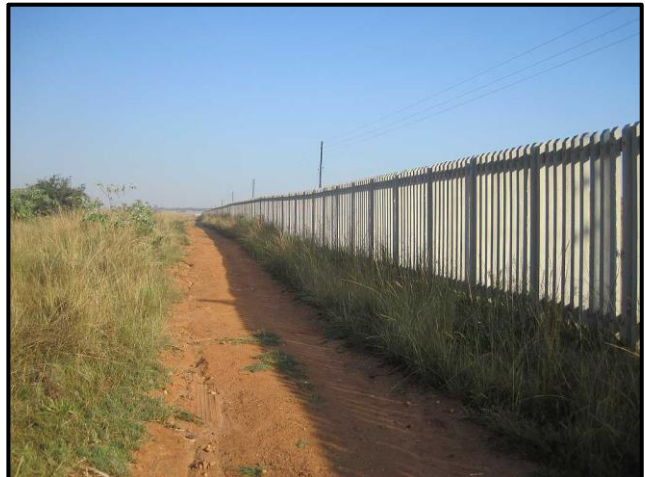
Figure 11. Cement palisade surrounding the site.
