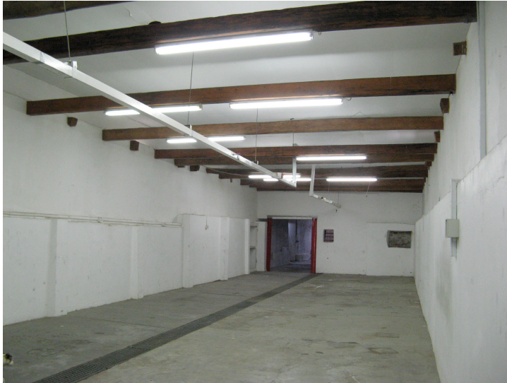
Figure 6: View of the extent of the 19 th century addition, facing eastwards.
