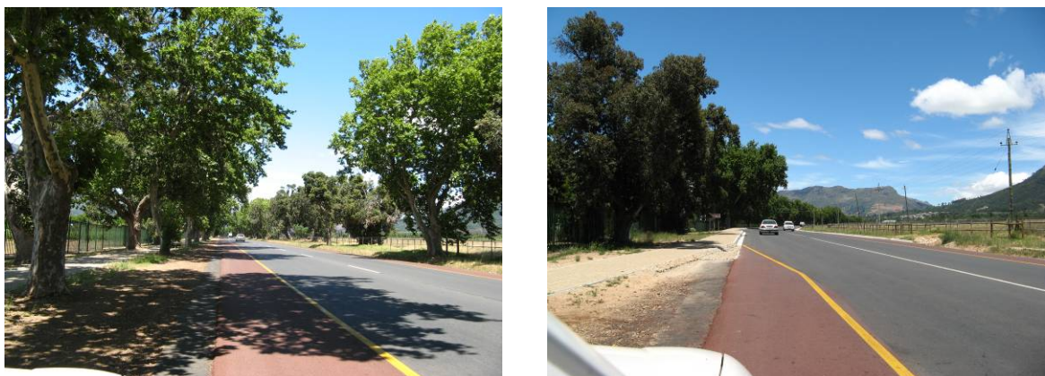
Plate 18: Views of the ongoing upgrade of the Helshoogte Road past Pniel and Boschendal. The visual bulk of the road is reduced through the use of tree lined pedestrian walkways. Cobbles as opposed to concrete are used to define kerbs and give a softer, less urban, feel to the road.
