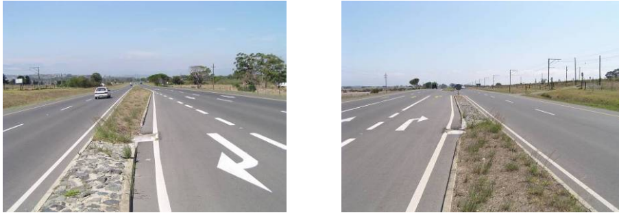
Plate 16: TR2/1 near Macassar, given as an example of the proposed road edge treatment for the proposed dual carriageway R310. The lack of vegetation along this section of the TR2/1 makes the road appear stark and harsh. This impression is emphasised by the powerlines running adjacent to this section of the TR2/1.
