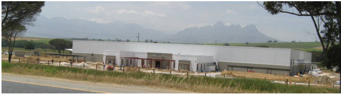
Plate 2: Bottling facility near Kompanjiesdrift road.
