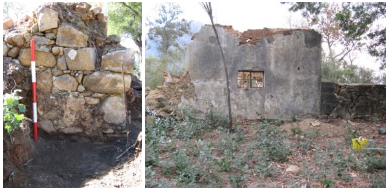
Figure 8: Details of the SE elevation of Cottage 1. Image on the left shows the construction style of the stone coursing. Image on the right shows the junction of the foundation of the cottage and that of the abutting stone kraal.
