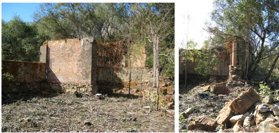
Figure 24: Brick enclosures viewed from the western extent.
