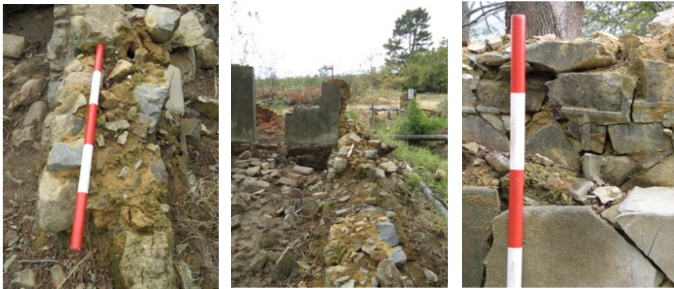
Figure 18: Stone boundary wall associated with Cottage 4.
