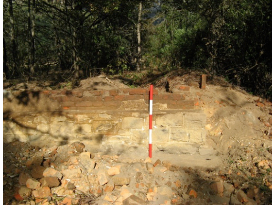
Figure 16: Mock pointing on Cottage 3. It appears as if the foundation consists of one course of stone. Mock pointing is visible on the remainder of the stone, which would have been exposed above ground level.
