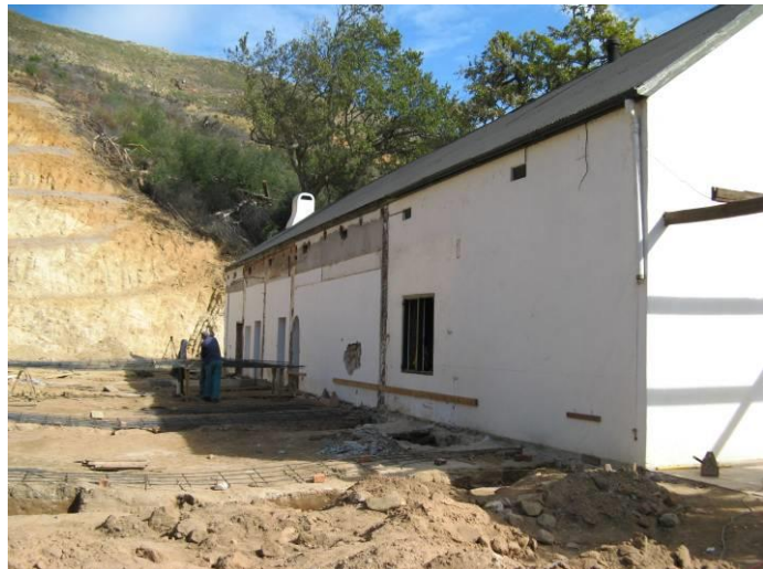
Figure 10: Present view of the southern flank of the dwelling. The 20 th century additions have been removed and extensive excavations have been undertaken for the new additions.
