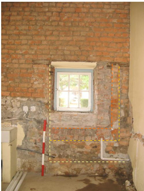
Figure 6: 18 th century casement window in kitchen, northern façade. An 18 th century lintel spans the dividing wall, suggesting a double casement was initially inserted in this position.
