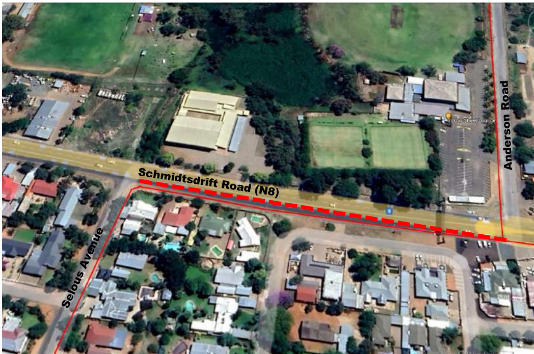
Figure 39: Aerial image of the Smidsdrift Road (N8) section of the route (dotted red section)
