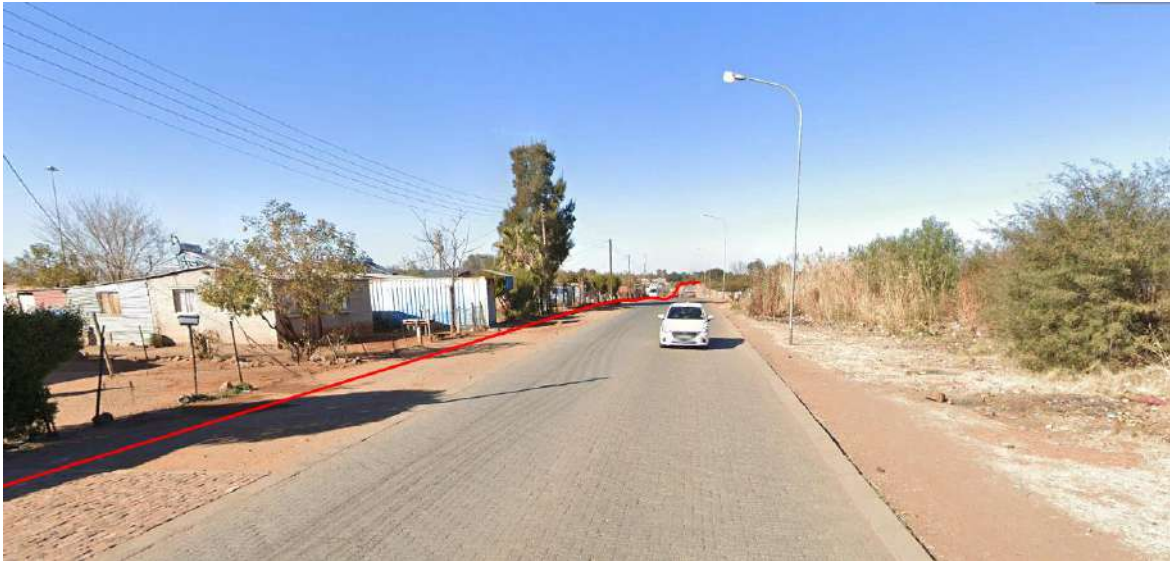
Figure 20: Line crosses Reserve Road where it runs in the sidewalk along the Single Residential properties of a residential area of Galeshewe
