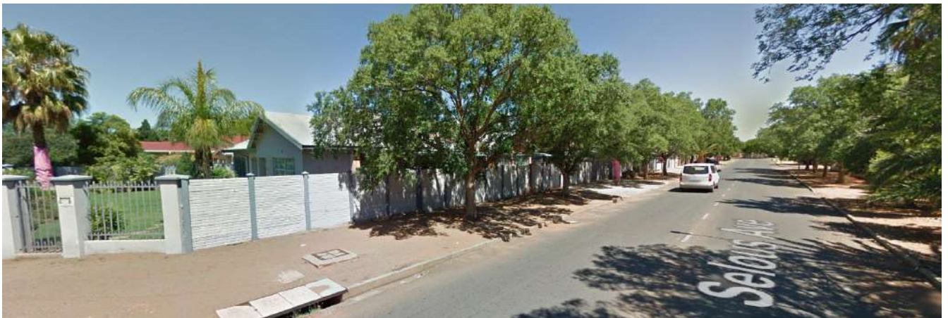
Figure 47: Streetscape in Selous Avenue close to the intersection with Smidtsdrift Road
