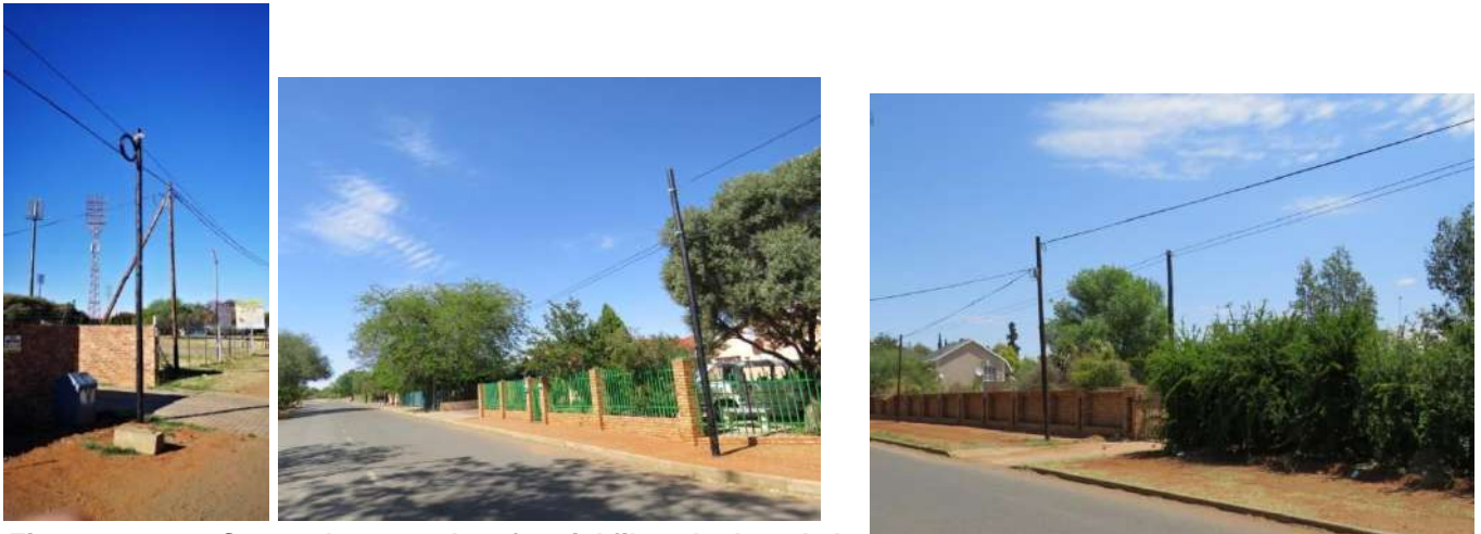
Figures 7 - 10: Some photographs of aerial fibre deployed elsewhere within the Municipal area
