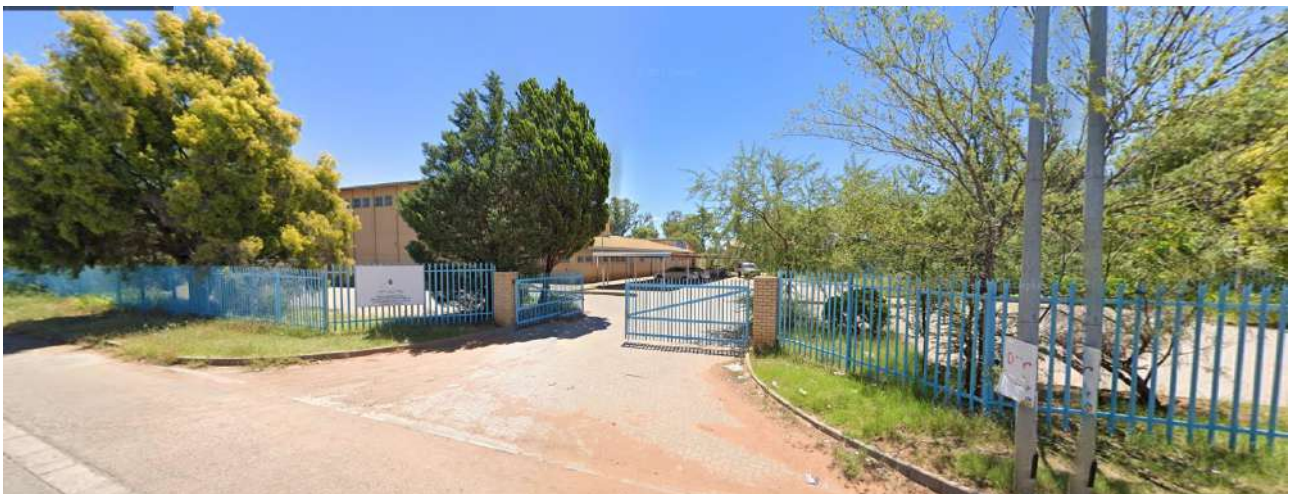
Figure 43: Jim Summers Hall (multi-purpose hall) on the northern side of Smidtsdrift Road
